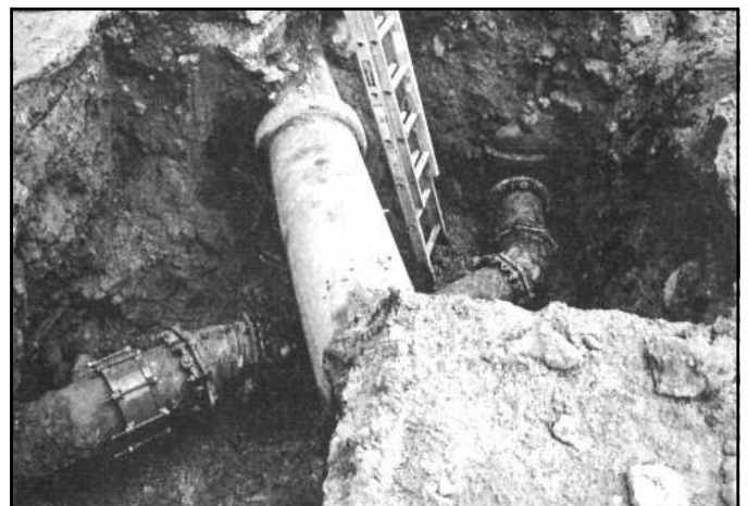
Haverlick Road – Water Main Replacement
