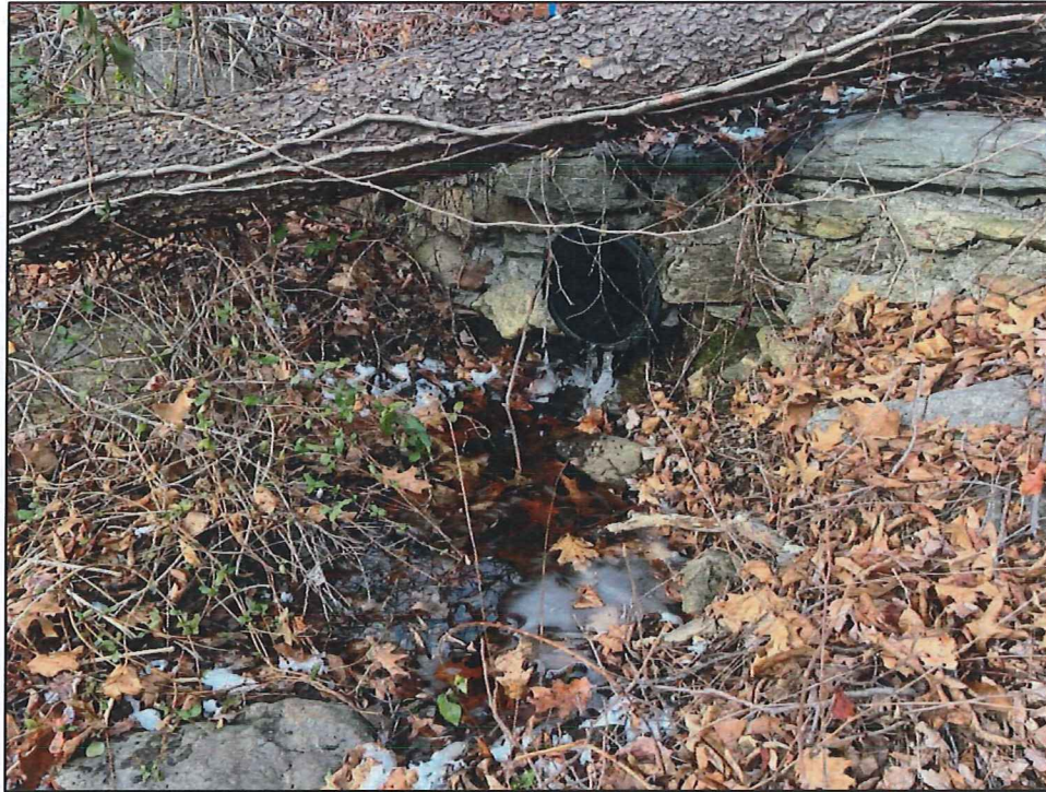
Figure C-9. View of Stream FR-S1 outlet flowing into Wetland FR-W1. Facing northwest.
