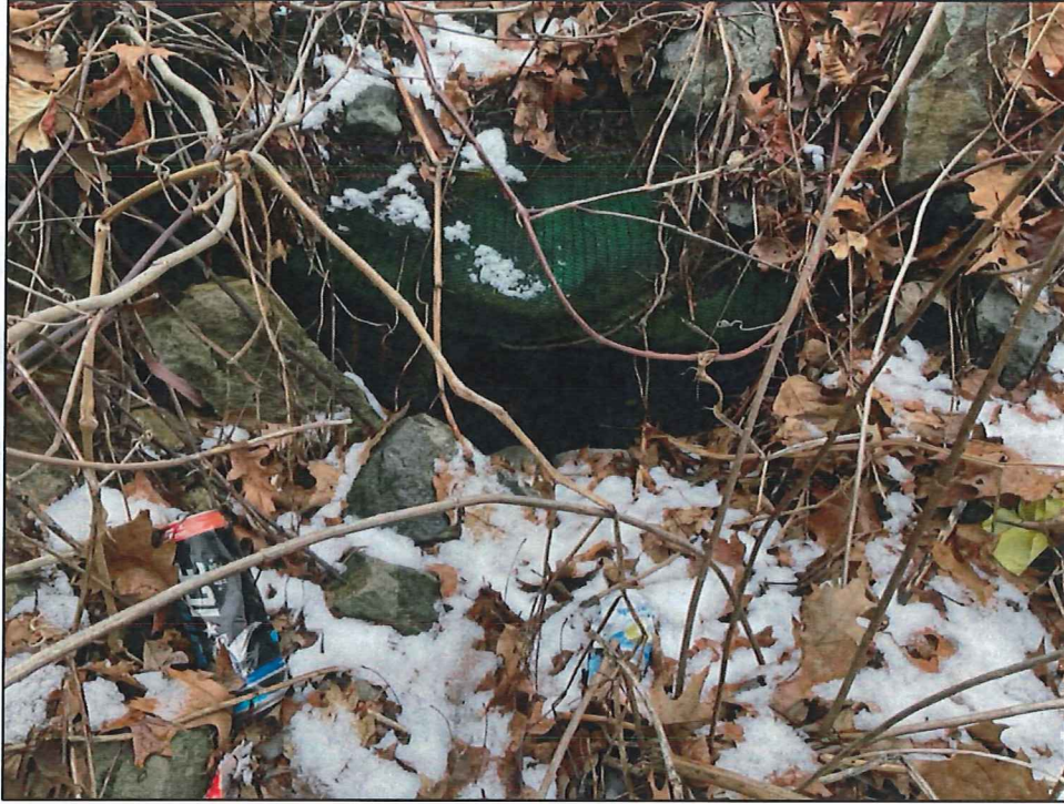
Figure C-5. View of Stream FR-S1 culvert inlet. Facing south.
