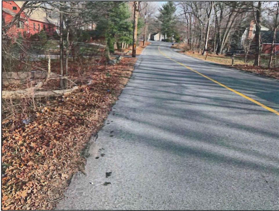
Figure C-7. View along Elm Street northern shoulder east of Stream FR-S1, where work is proposed. Facing east.
