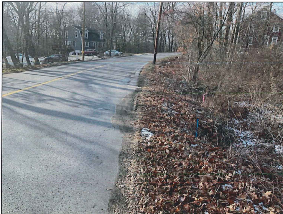
Figure C-6. View of Elm Street northern roadway shoulder west of Stream FR-S1. Facing west.
