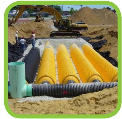
StormTech Isolator Row PLUS with Overflow Spillway (not to scale)
