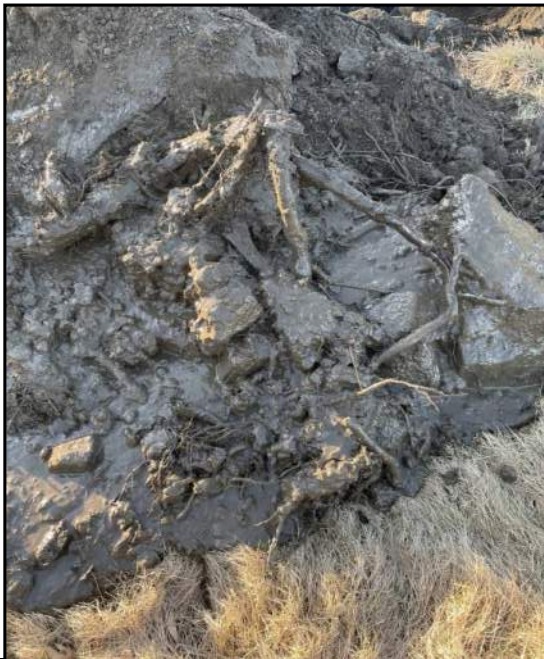
TP-106 spoils pile detail - organics
