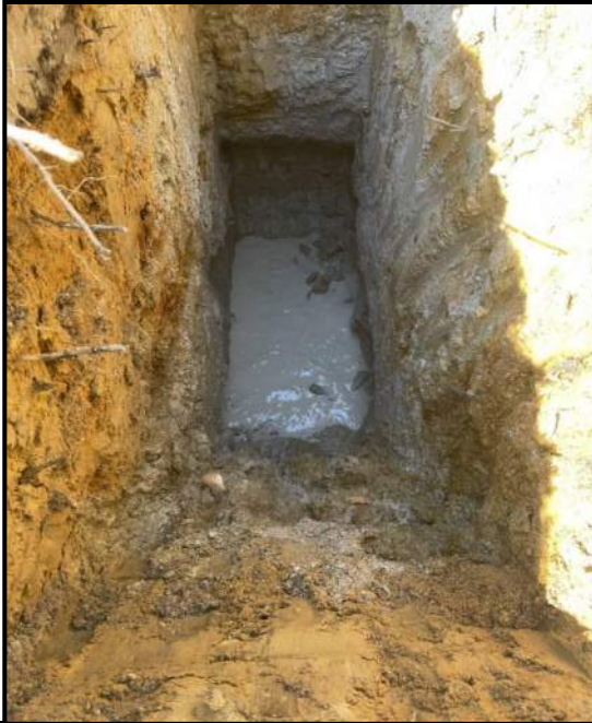
Test pit TP-115
