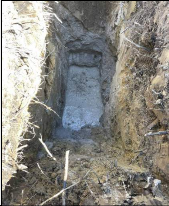
Test pit TP-116
