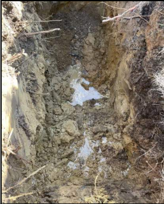
Test pit TP-110
