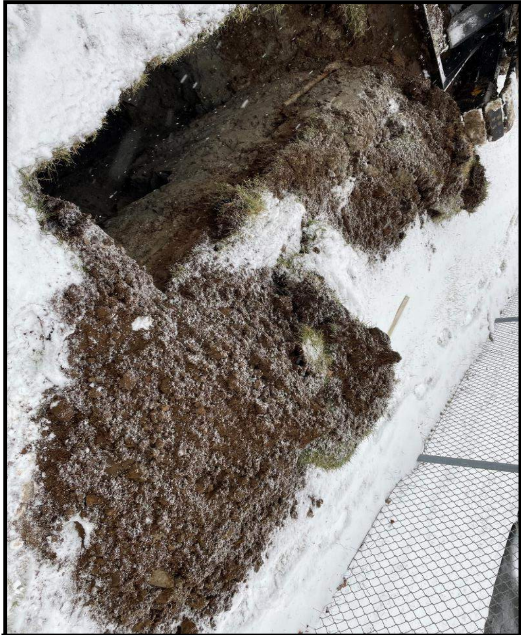
Test pit TP-101 and topsoil spoils pile
