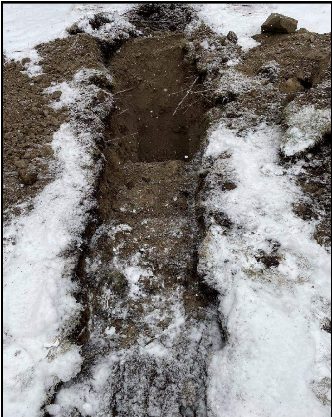
Test pit TP-103
