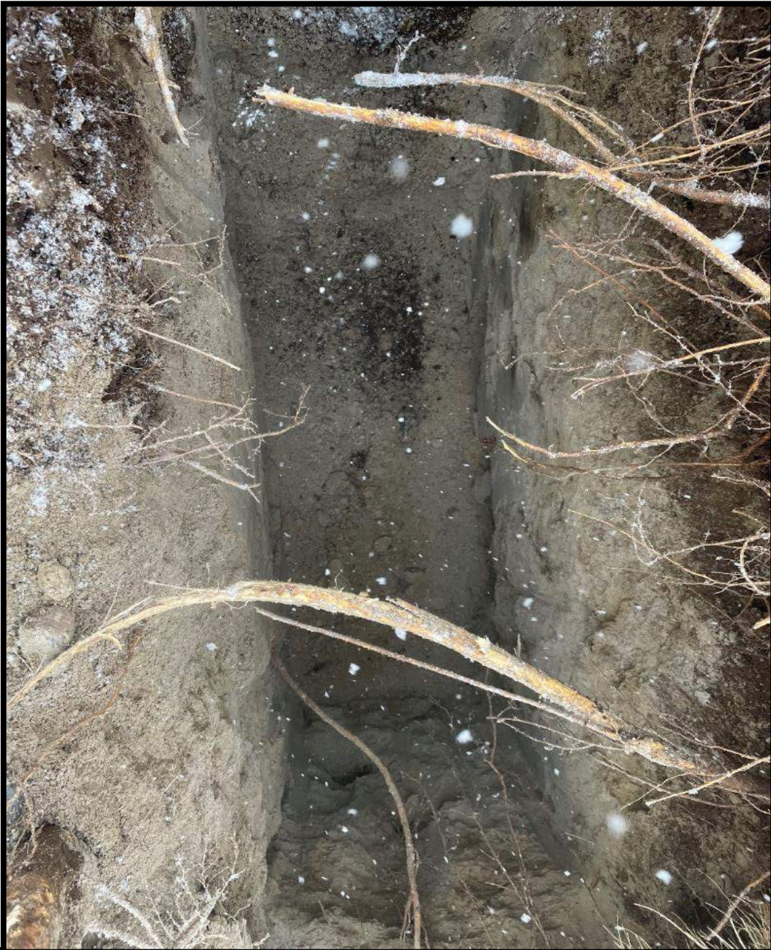
Test pit TP-104
