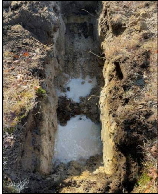
Test pit TP-111
