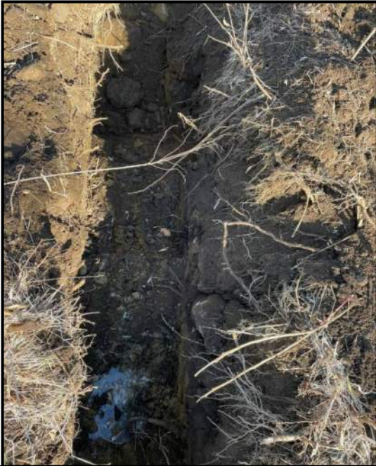
Test pit TP-111
