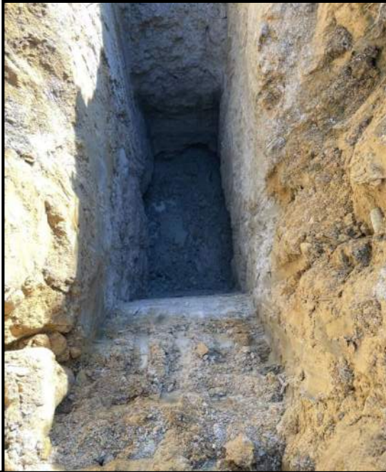
Test pit TP-114
