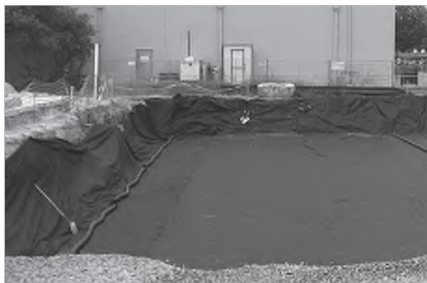
Place non-woven geotextile over prepared soils and up excavation walls. Install underdrains if required.
