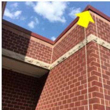
Roof-Wall Intersection Air Sealing – the exterior flashing and finishes at the roof-wall intersection are not constructed to stop air leakage (Keller/ Sullivan School).
