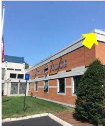
Roof-Wall Intersection Air Sealing – the exterior flashing and finishes at the roof-wall intersection are not constructed to stop air leakage (Police Station).
