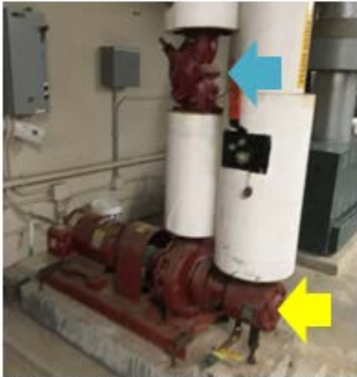
Valve & Fitting Insulation – the suction diffuser (yellow) and strainer (blue) are not insulated which is leading to unnecessary distribution losses (Keller Sullivan School).
