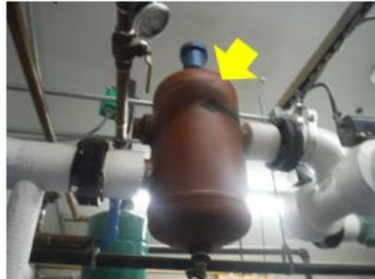
Tank Insulation – the air separator tank represents a large surface area in the heating distribution which if continued to left uninsulated will result in distribution losses (Municipal Building).
