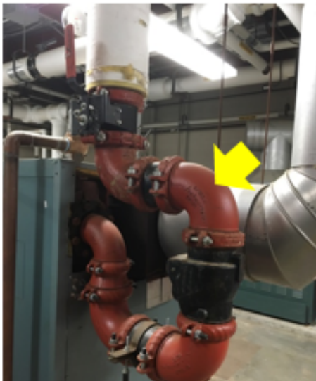
Pipe Insulation – Victaulic pipe insulation was removed. Exposing pipe to unconditioned boiler room is leading to unnecessary distribution losses (Keller/Sullivan School).
