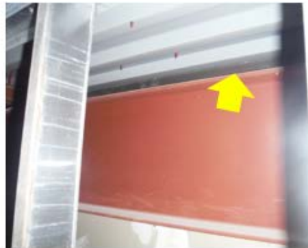
Roof-Wall Intersection Air Sealing – gaps at the interior of the roof-wall intersection combine with the unsealed exterior flashing and finish details to allow unwanted infiltration/ exfiltration (Municipal Building).
