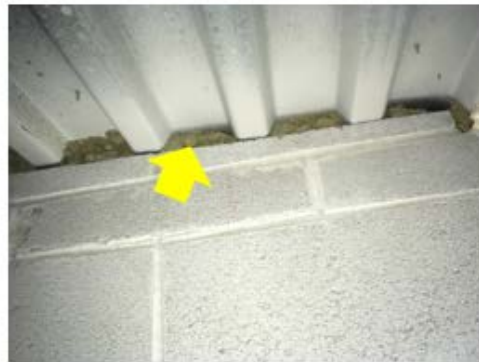
Roof-Wall Intersection Air Sealing – fiberglass was used to fill gaps between the roof and wall framing components. Fiberglass is an air permeable material that needs to be covered with an air barrier to avoid further air leakage at the roof-wall intersection (Keller Sullivan School).
