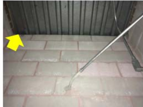
Roof-Wall Intersection Air Sealing – gaps between the roof deck and the wall framing are pathways for unwanted infiltration/ exfiltration (Police Station).
