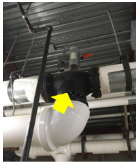
Valve & Fitting Insulation – the 3-Way valve in the distribution system is a tricky component to insulate. The large uninsulated surface needs to be wrapped in order to reduce distribution losses (Keller Sullivan School).
