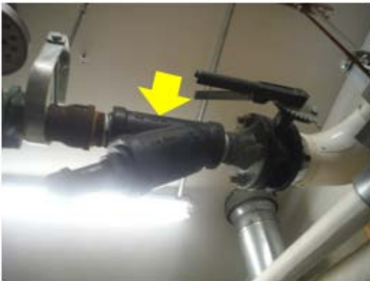
Valve & Fitting Insulation – the strainer is uninsulated which is leading to unnecessary distribution losses (Municipal Building).
