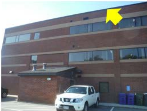
Roof-Wall Intersection Air Sealing – the exterior flashing and finishes at the roof-wall intersection are not constructed to stop air leakage (Municipal Building).
