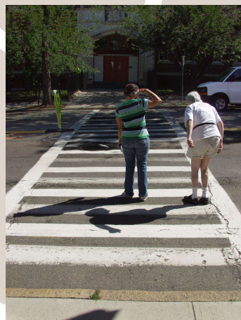
Lack of curb ramps and curb extensions
