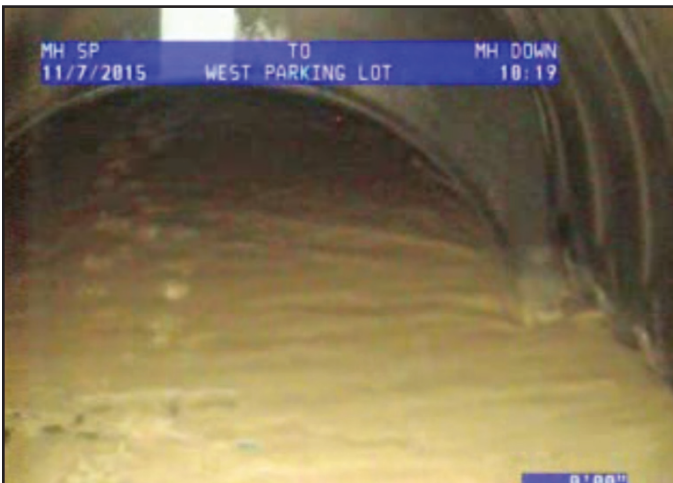
SEPARATOR ROW: Separator Row prior to cleaning
