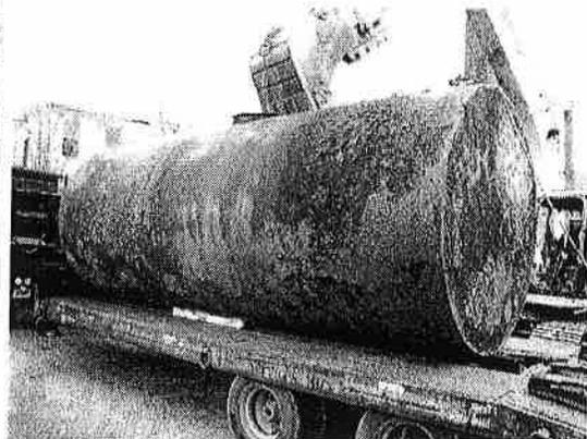
**Photo 12:** View of the northern side of the UST as it was placed on a trailer for offsite disposal.
