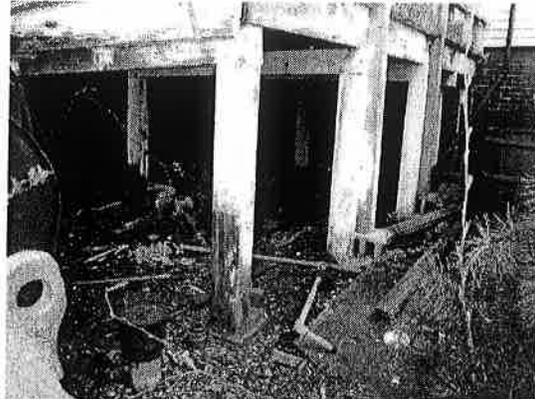
**Photo 2:** Close-up view of the UST area, looking east. Concrete tank pad was covered with debris. UST fill pipe (lower left) and vent pipe (upper right) are visible.
