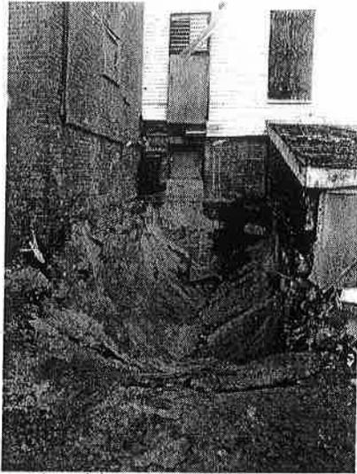
**Photo 13:** View of the tank grave following UST removal, looking east.
