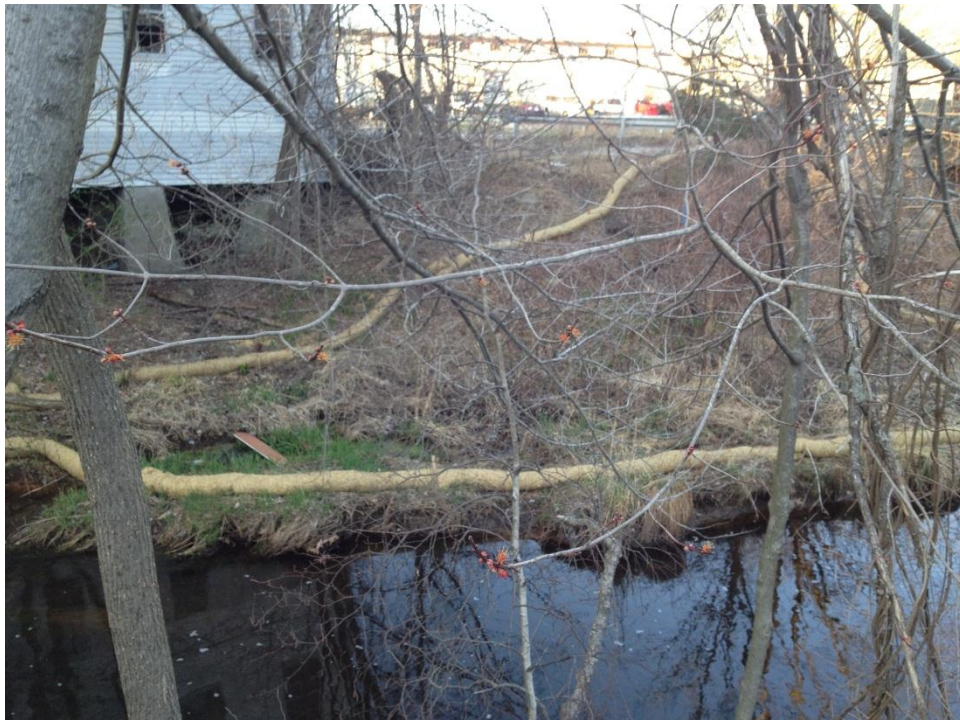
Erosion controls installed along Mine Brook
