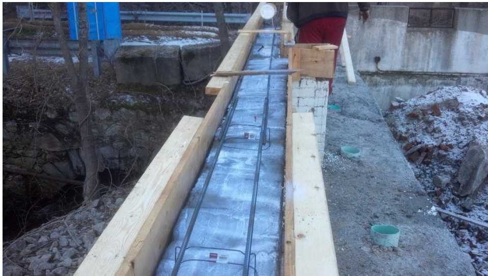
The foundation wall was capped with a poured concrete cap
