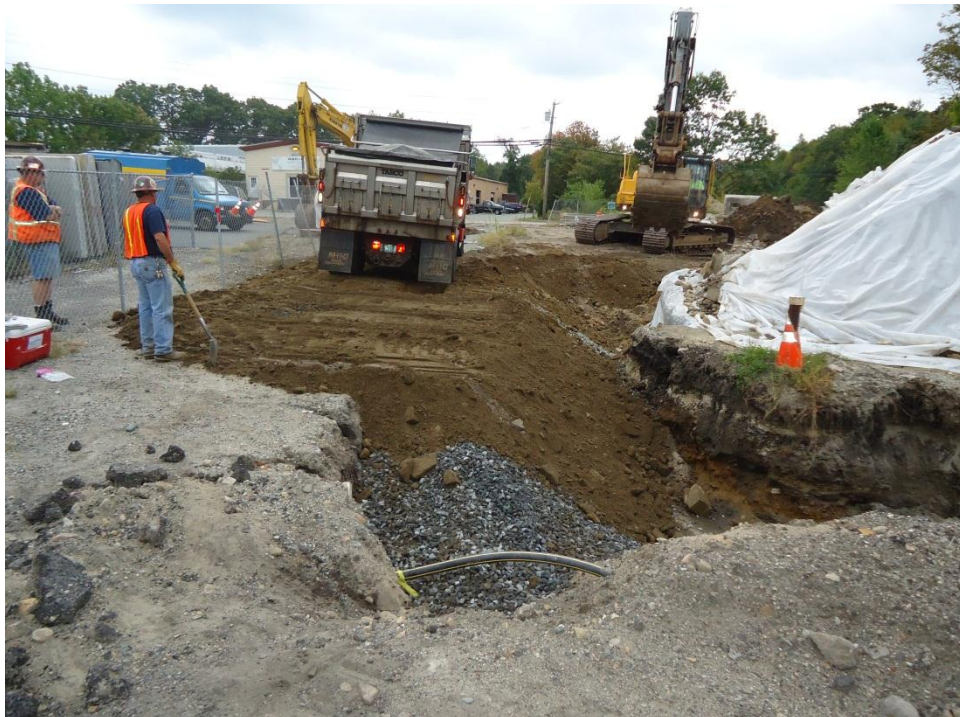
Backfilling the northwest excavation area
