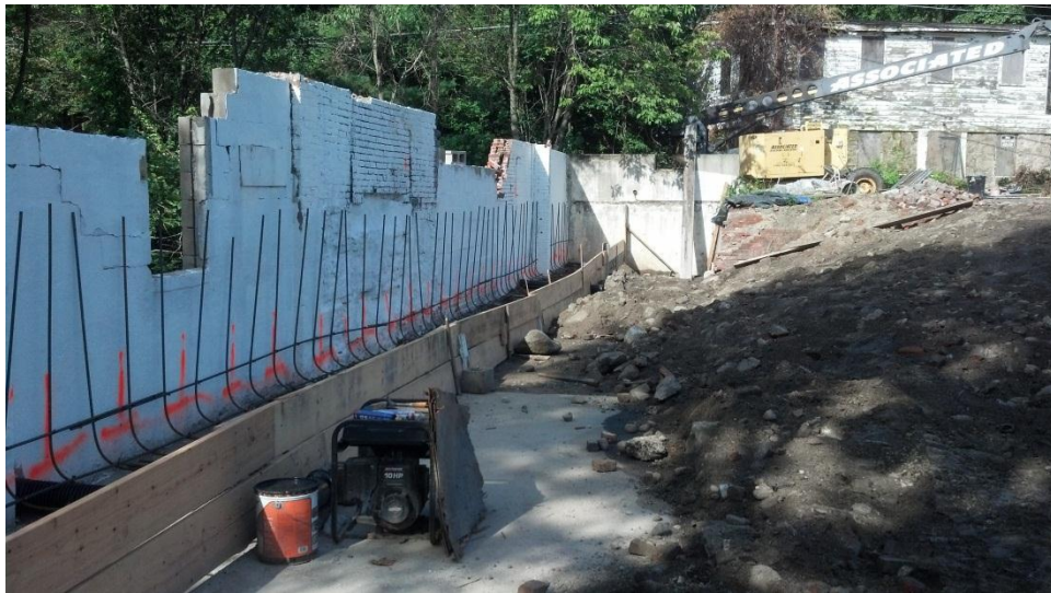
Installation of the concrete form work for the gravity wall
