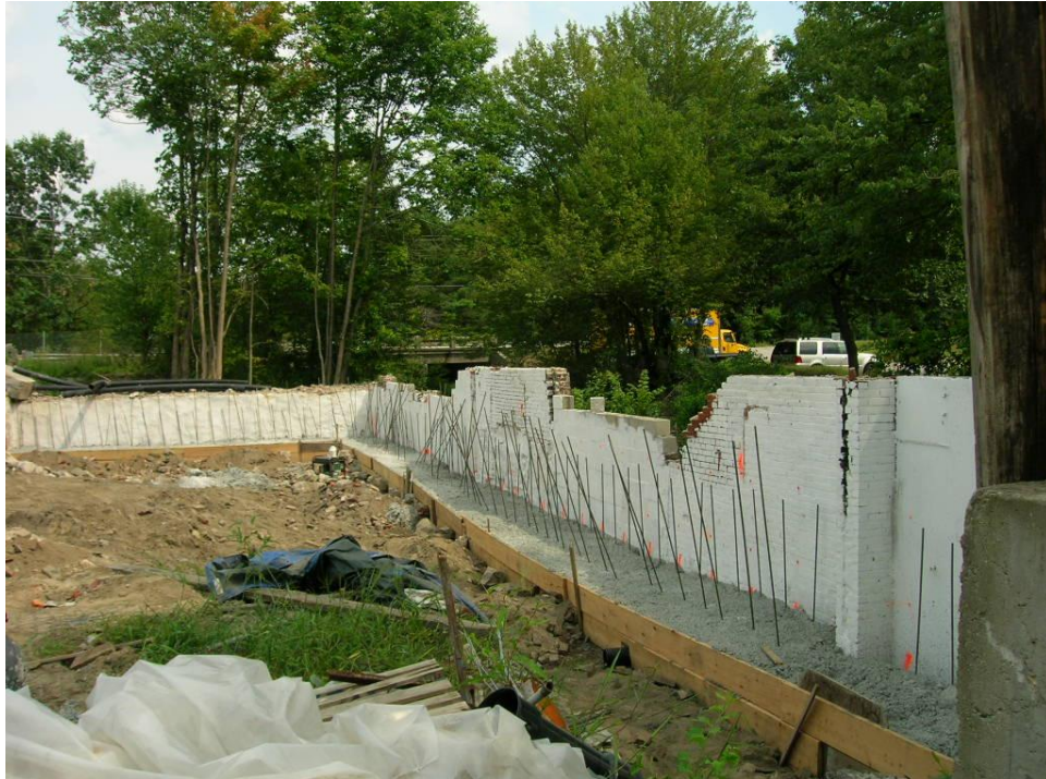
The cast-in-place concrete gravity wall behind the foundation façade
