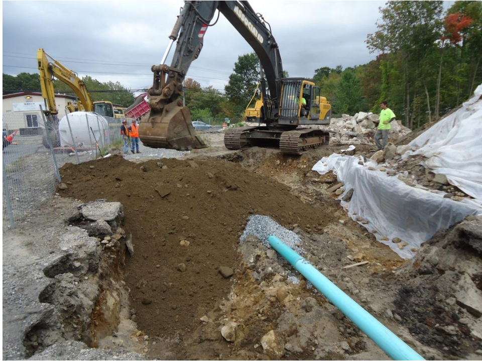
The repaired sewer line, which limited the excavation along the northern property line
