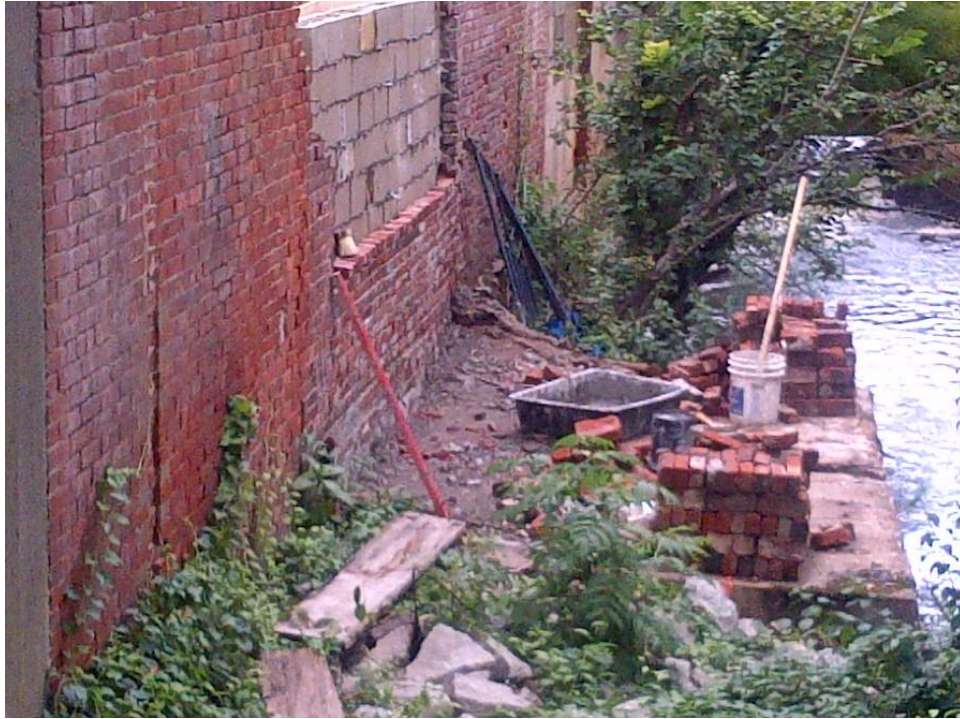
Restoration of the brick masonry wall façade
