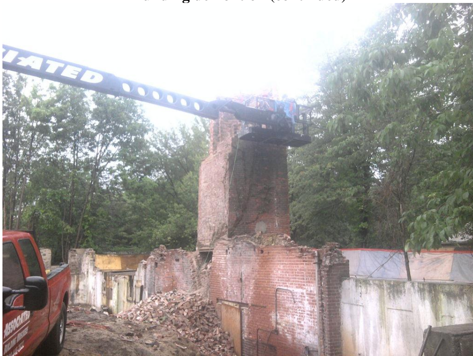
The chimney was demolished by hand and bricks were pulverized for fill
