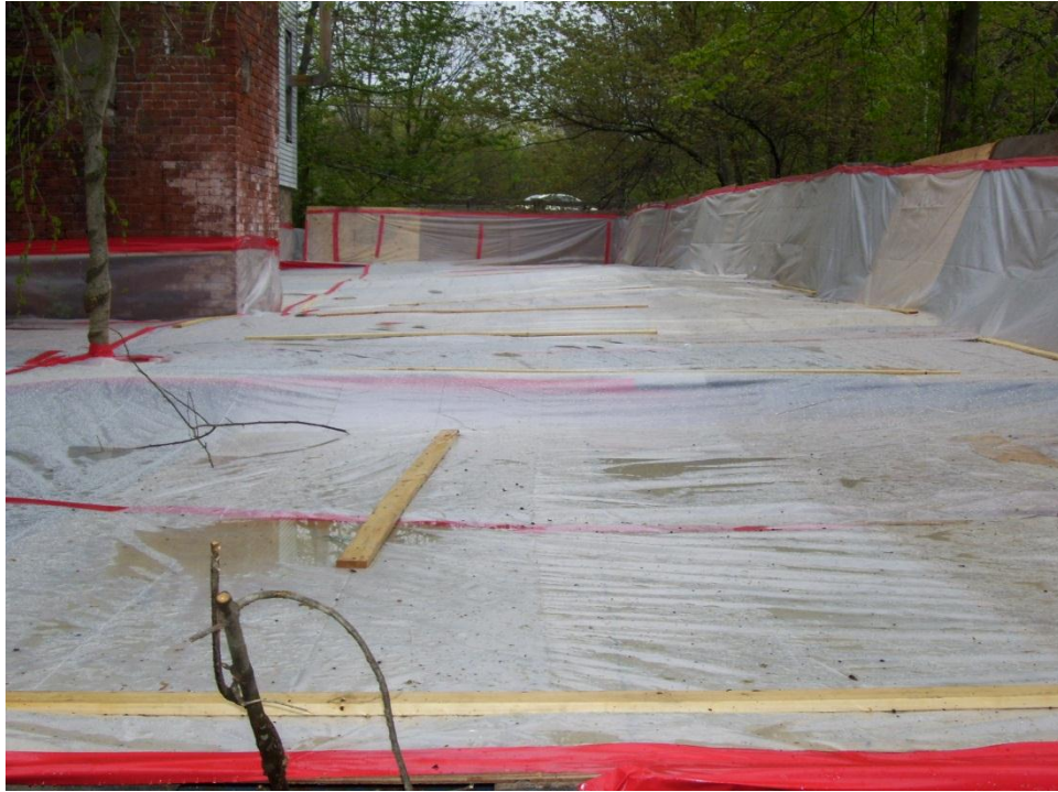
A scaffolding structure was used to prevent falling debris from impacting wetlands
