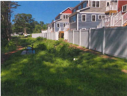
View showing stable drainage swale and walking path in southern portion of site.
