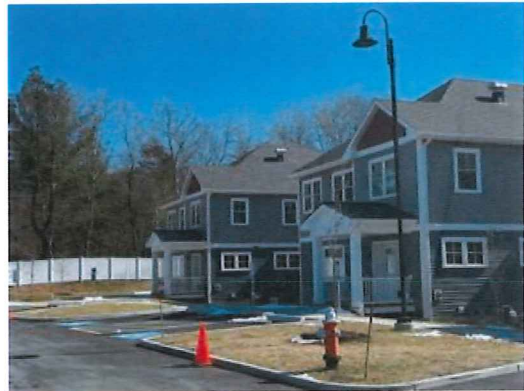
View showing stable lawn areas and pavement at residence buildings in southern portion of site.
