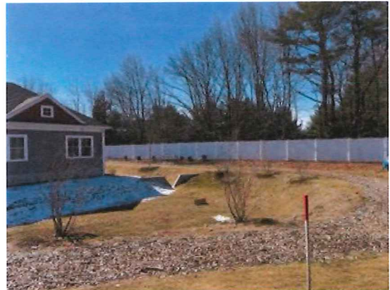
View showing stable infiltration basin in northwestern portion of site.
