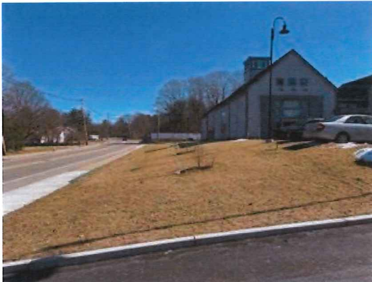
View showing stable front lawn along Washington Street.
