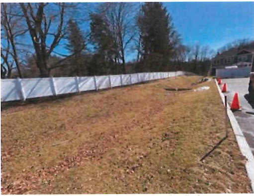
View showing stable infiltration basin in eastern portion of site.
