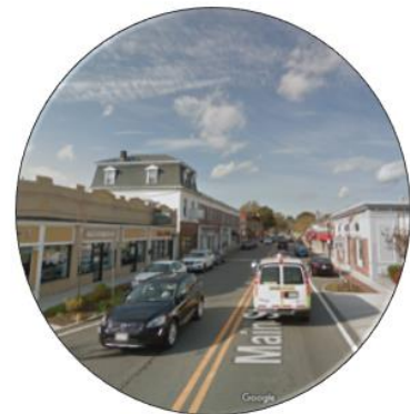
Figure 8: View up Main Street showing continuous streetwall.
