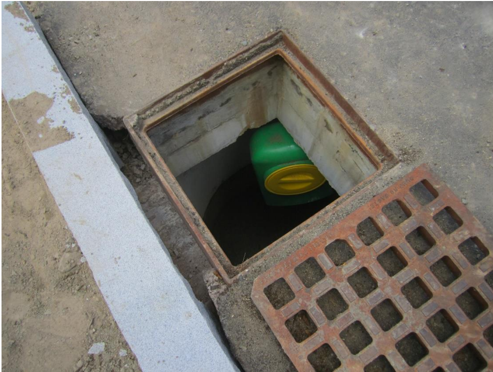
Typical hood installation
