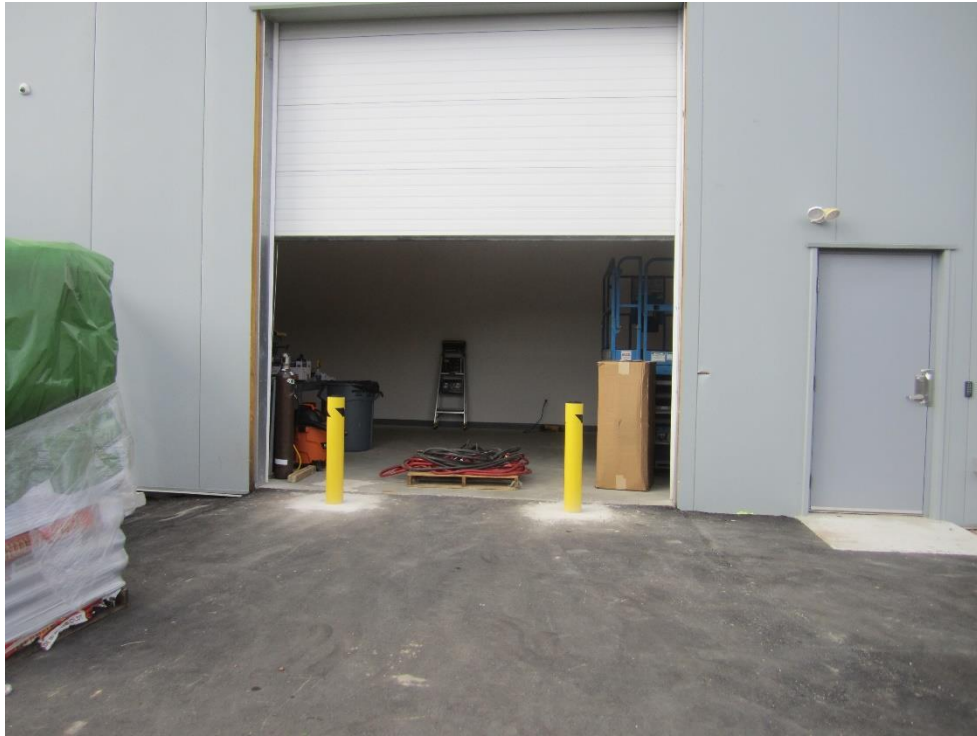
Bollard installation at access door
