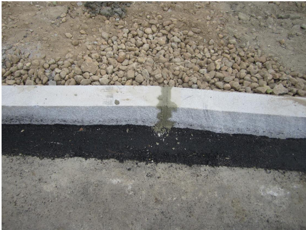
Recently pointed curb
