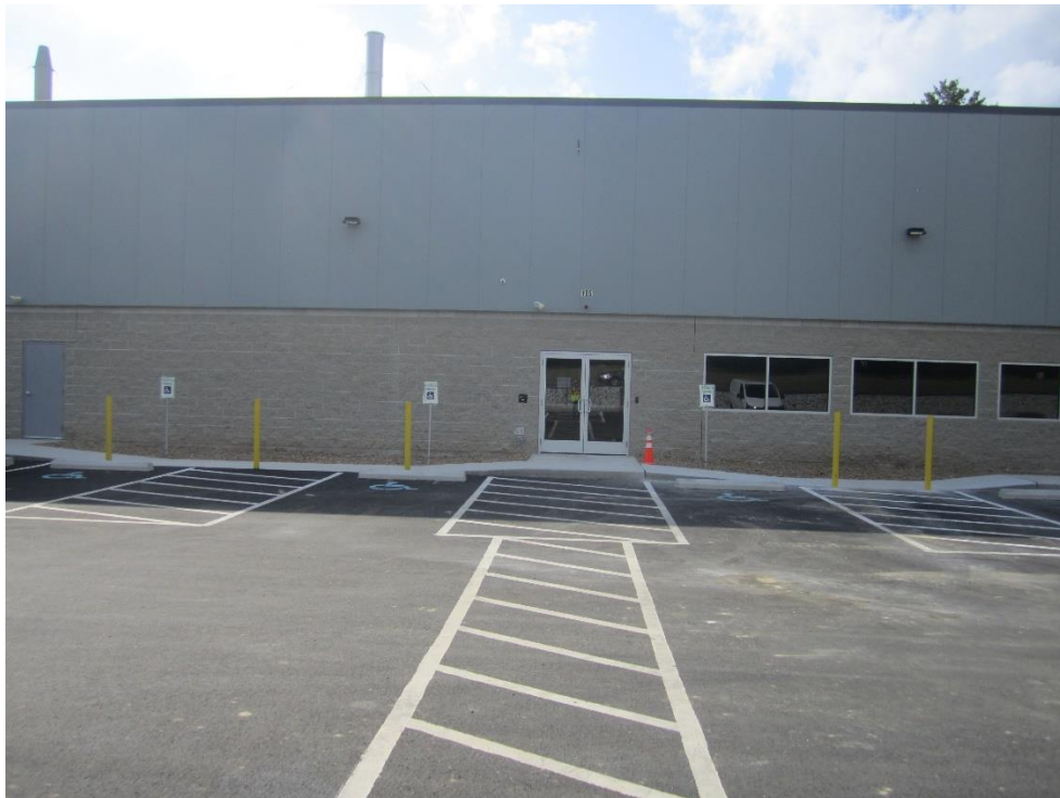
Accessible parking with required aisles, ramps, and permanent signage
