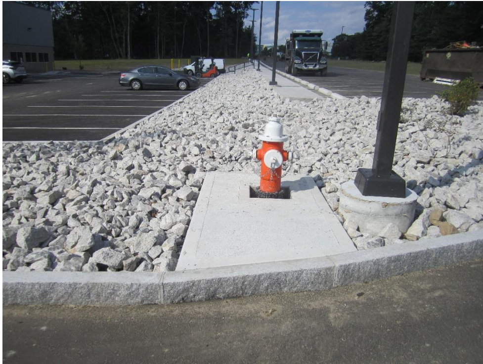
Concrete access pad installed around hydrant
