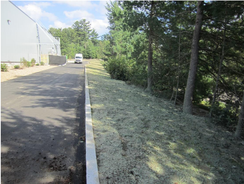
Typical final grading behind curb
