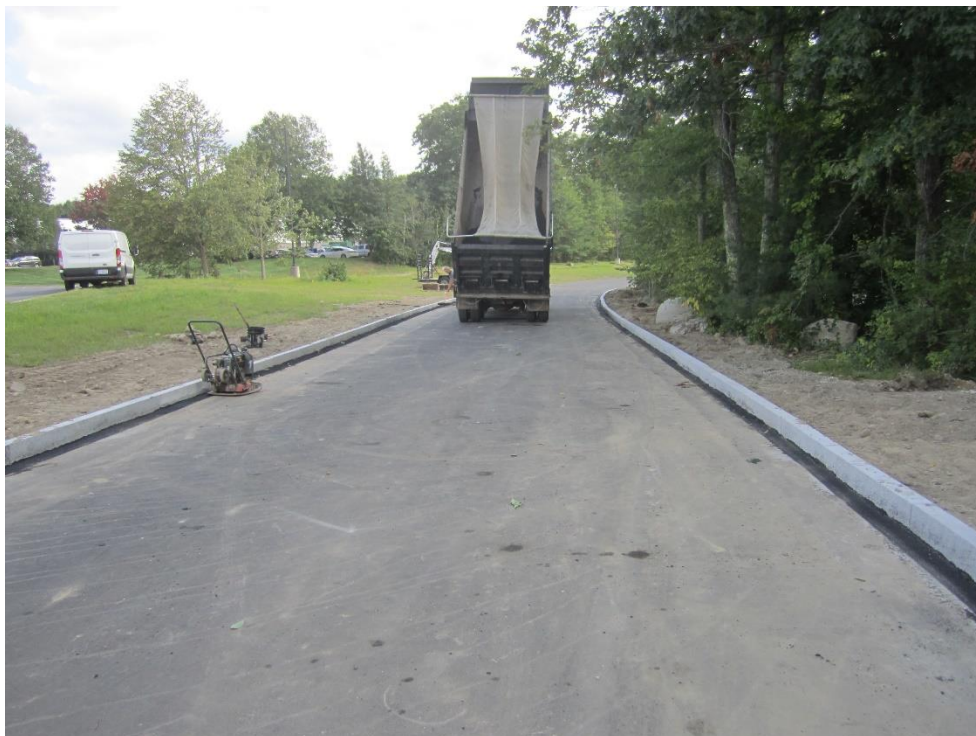
Typical curb installation near site entrance
