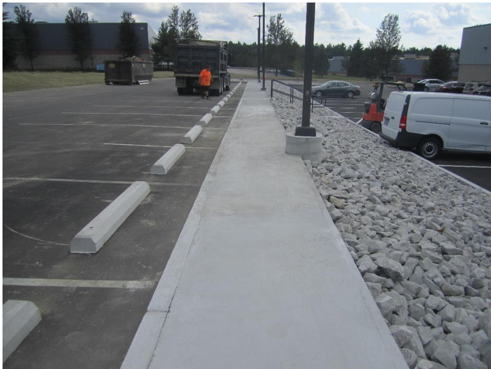
Typical 48" sidewalk (excluding curb) with adjacent car stops
