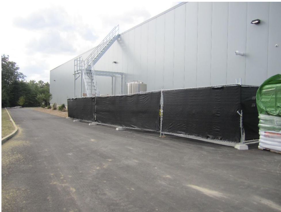
Temporary fencing installed around dumpsters and roof access stairs
