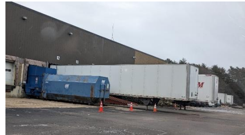
View of loading bays at 8:00 AM.
