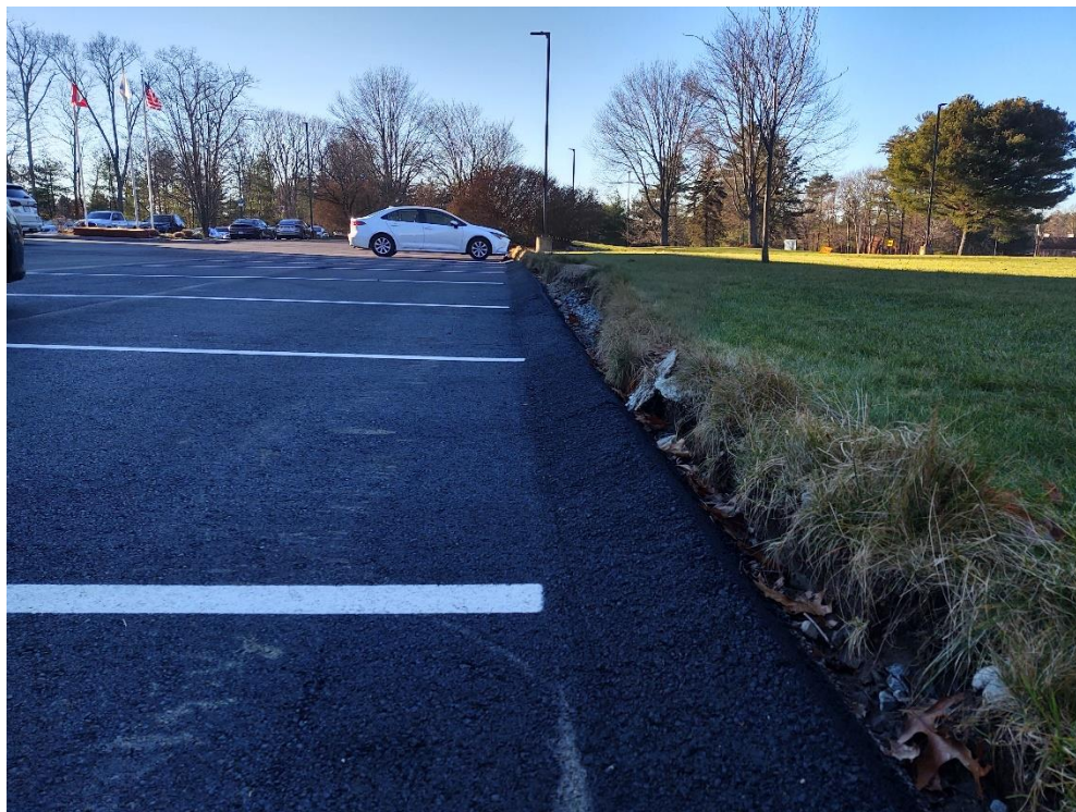
Typical berm installation (replaces existing)
