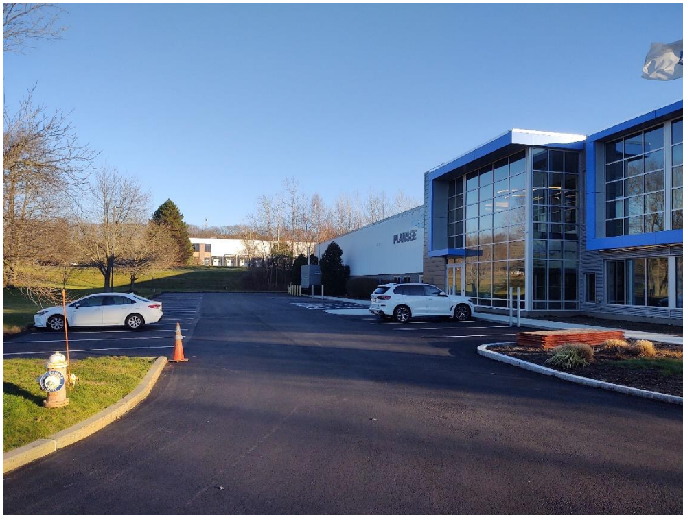
Typical paved parking area
