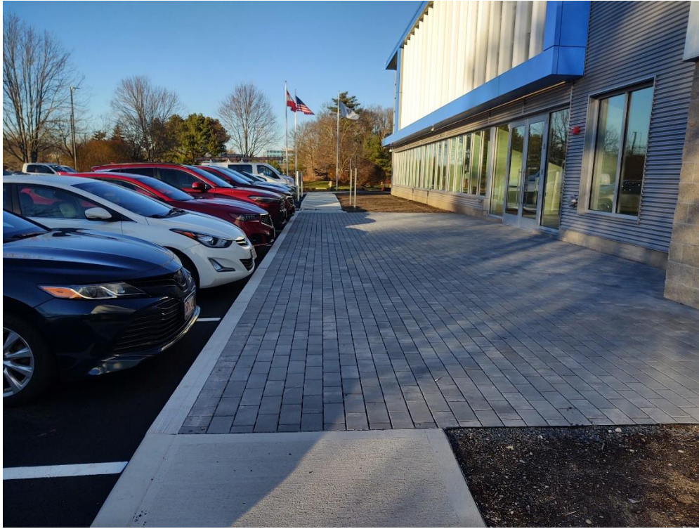
Pervious paver plaza area. Granite bollards to be installed 12/15/23
