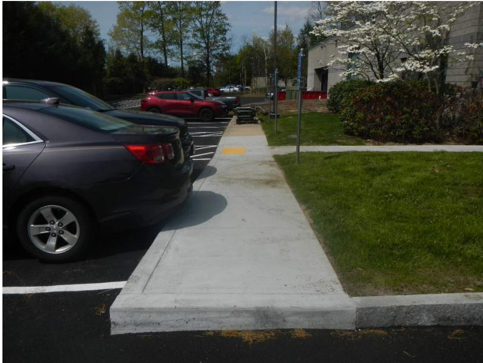
New concrete sidewalk (photo taken 5/9/23)
