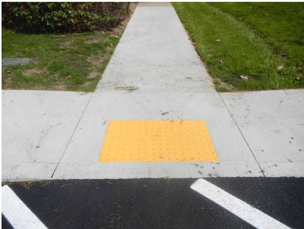
Accessible ramp (photo taken 5/9/23)
