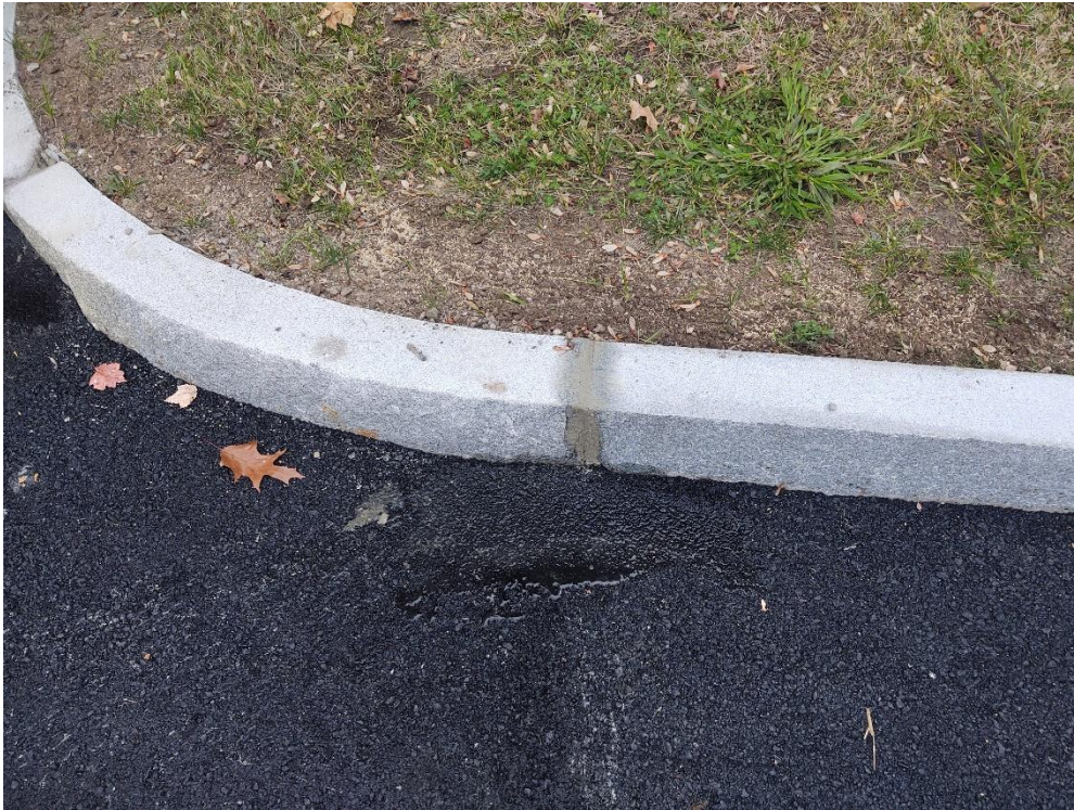
Pointed granite curb
