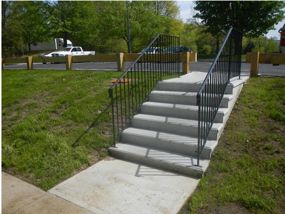
Installed concrete stairs and handrails (photo taken 5/9/23)
