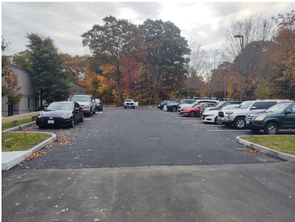
New parking area
