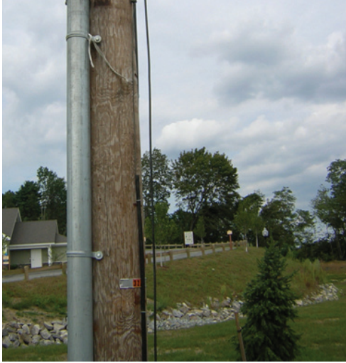
Riser Pole Bonding Rigid Galvanized Steel. Bond higher than 8' and at least 6" from top.
