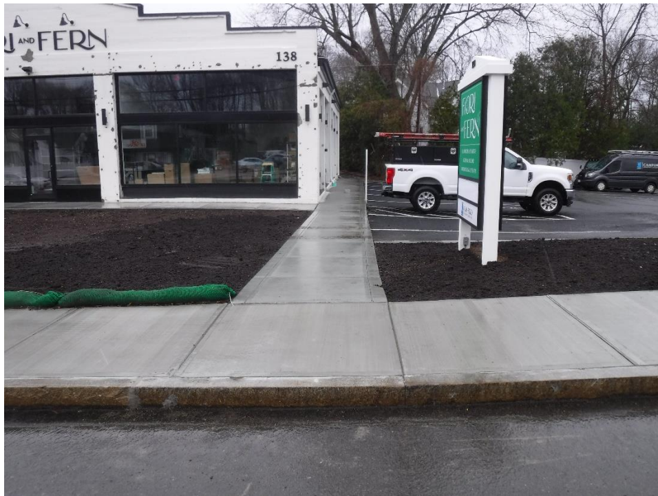
Accessible route from public sidewalk to building
