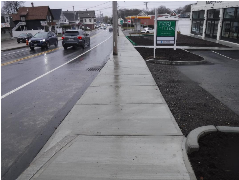
New concrete driveway apron
