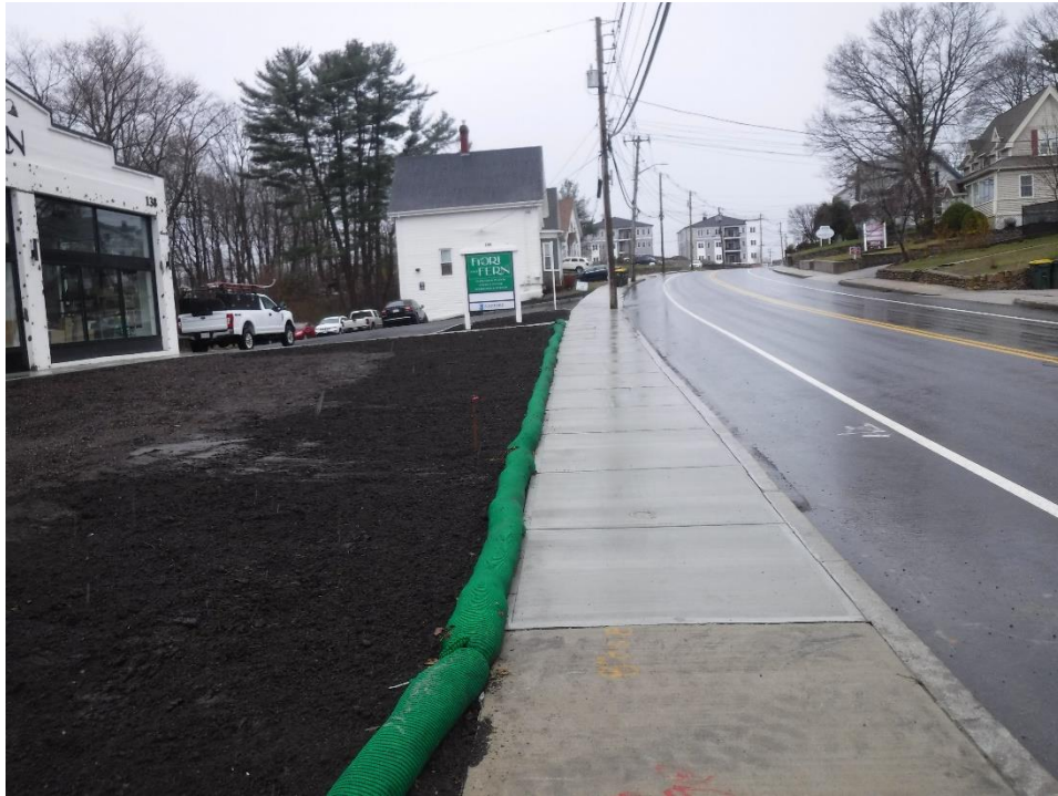
New sidewalk along E. Central frontage
