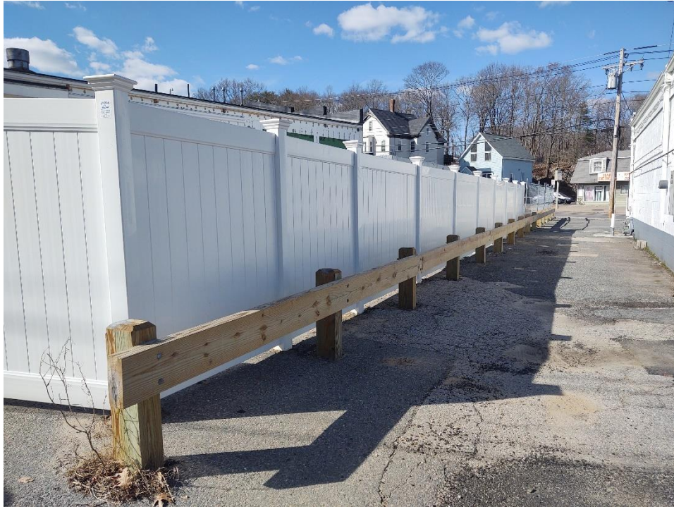
Wooden guardrail and fencing along west side of site (photo 3/18/24)
