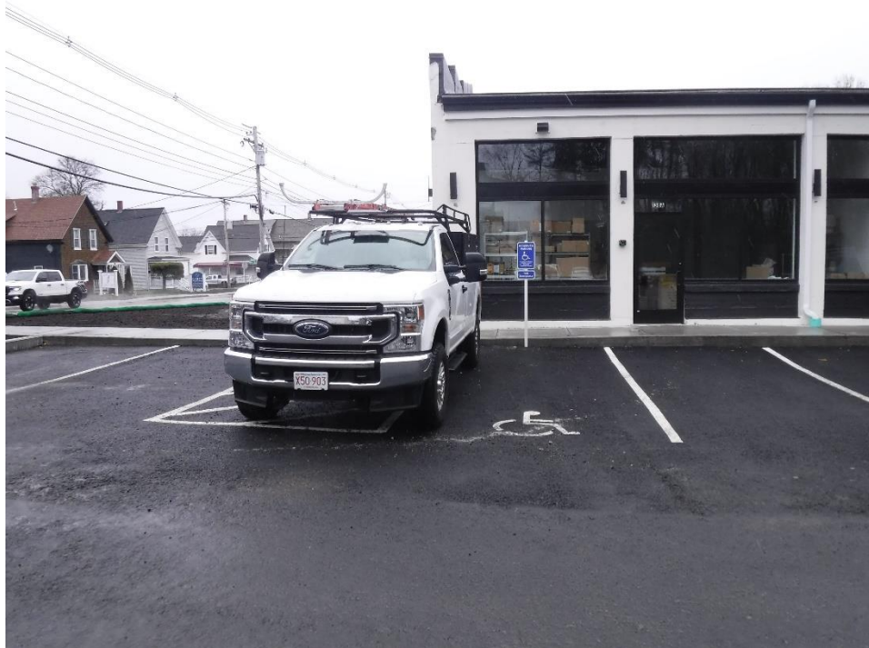
Accessible parking space and signage (ramp provided at rear of vehicle)
