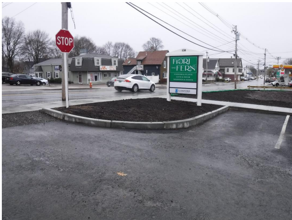
Typical curb installation and site signage
