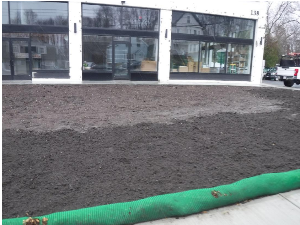
Loam placed above subsurface infiltration system
