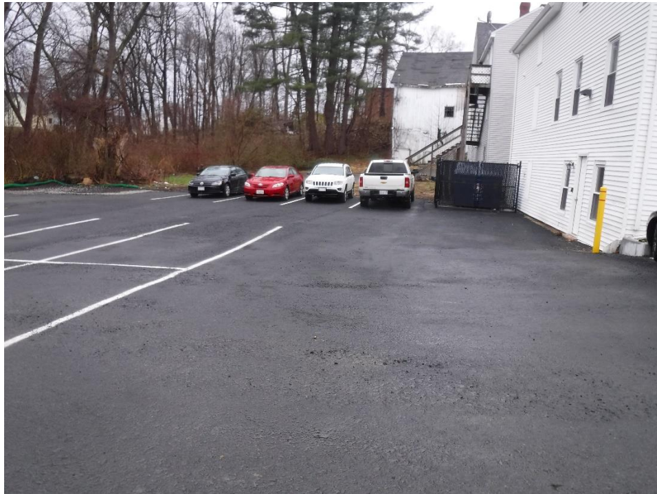
Bollard adjacent to building and trash enclosure in background
