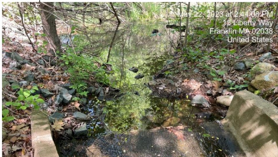
Figure 3: View of riprap lined IVW from concrete pipe outlet, facing north.
