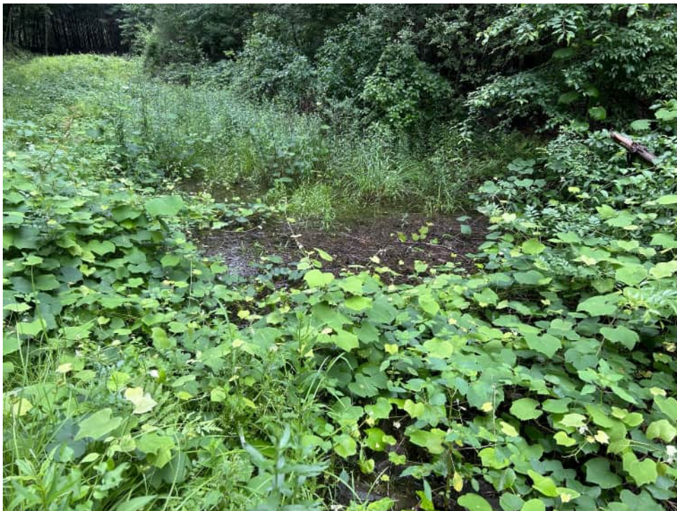
View of the ponding upgradient of the IVW—facing north.
