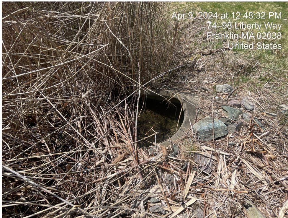
Figure 6: Outlet of drainage pipe entering offsite detention pond.
