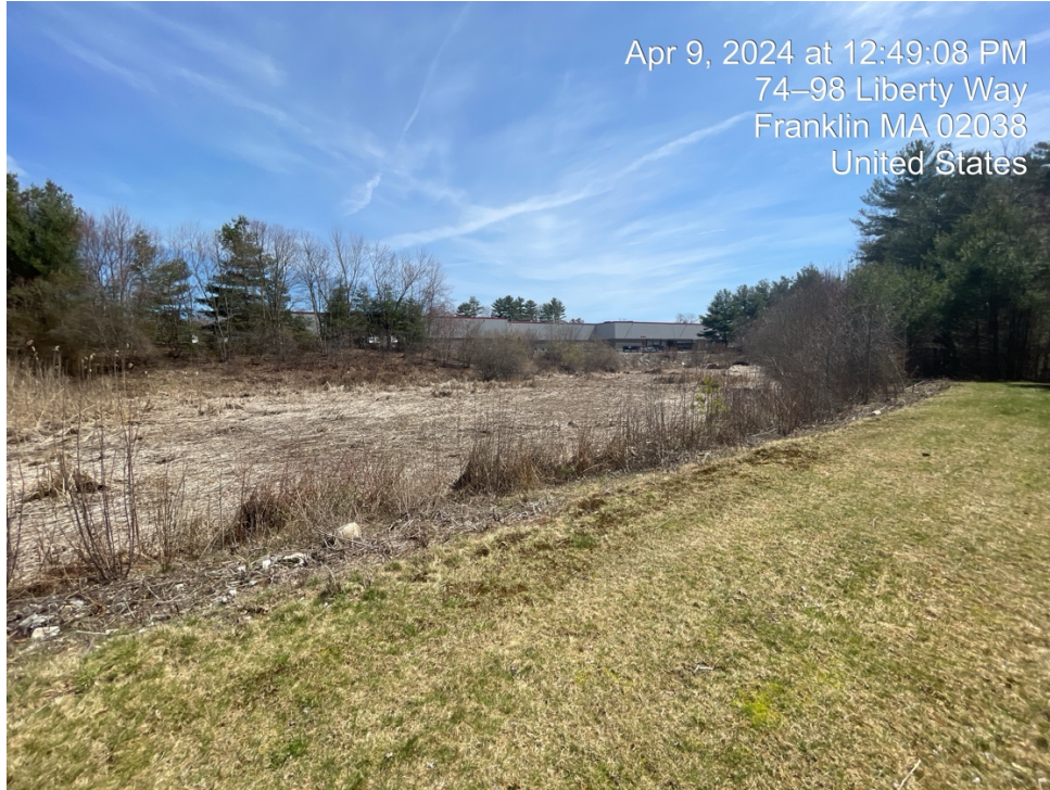
Figure 4: View of offsite detention pond facing southeast.
