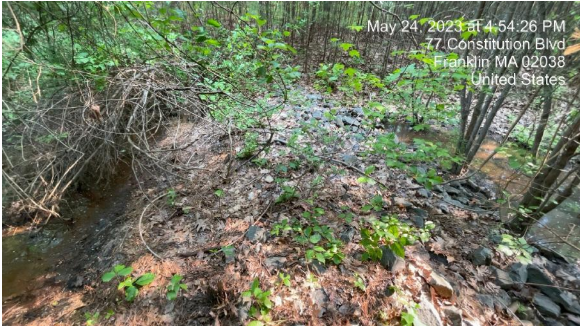
Figure 6: Unmaintained riprap breaker interrupting stormwater ditch.
