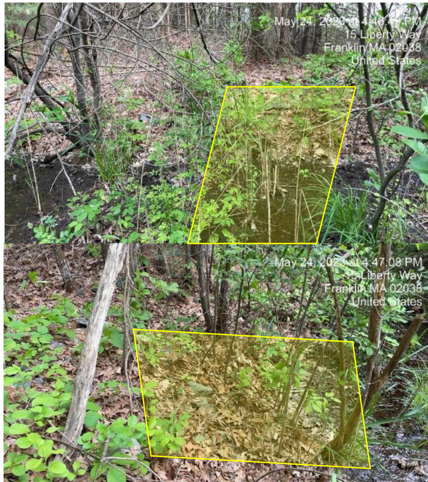
Figure 10: Two photos showing approximate location of proposed supplemental riprap in yellow.
