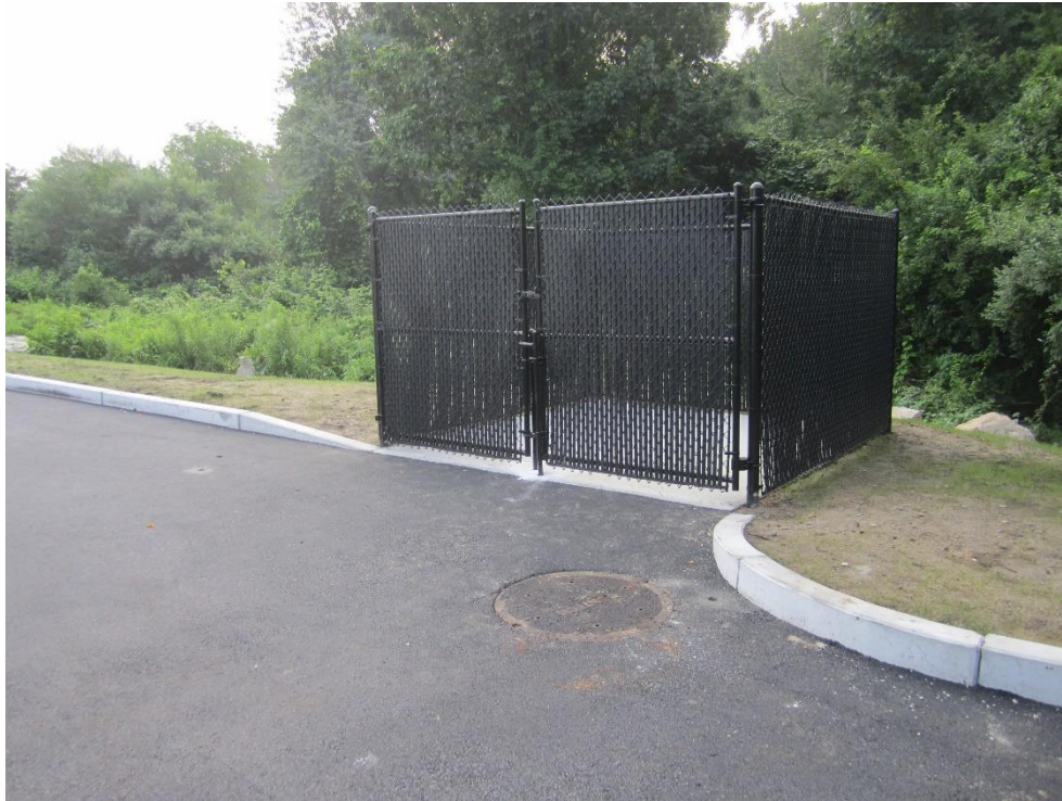
Dumpster pad and enclosure
