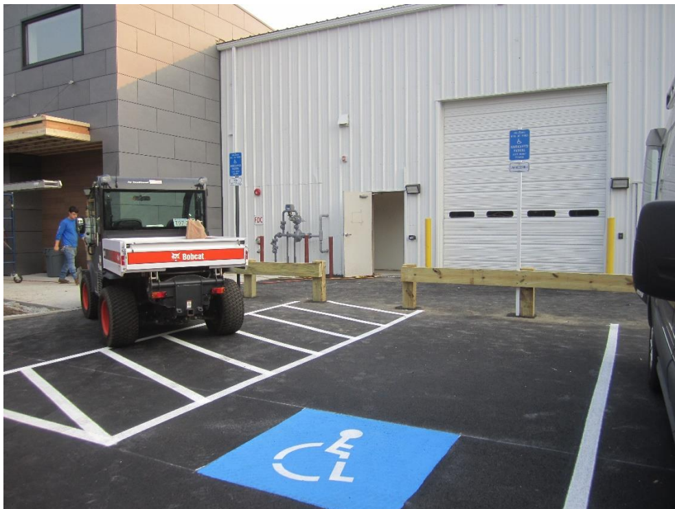
Typical accessible parking space
