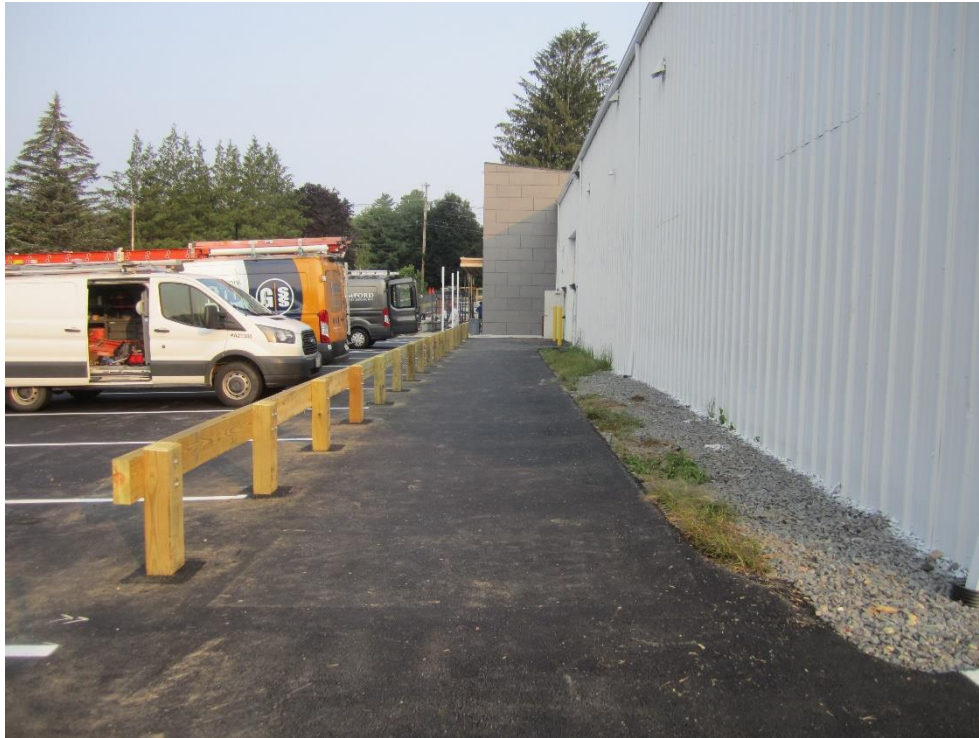
Bituminous walkway to building with wooden guardrail separating from parking spaces
