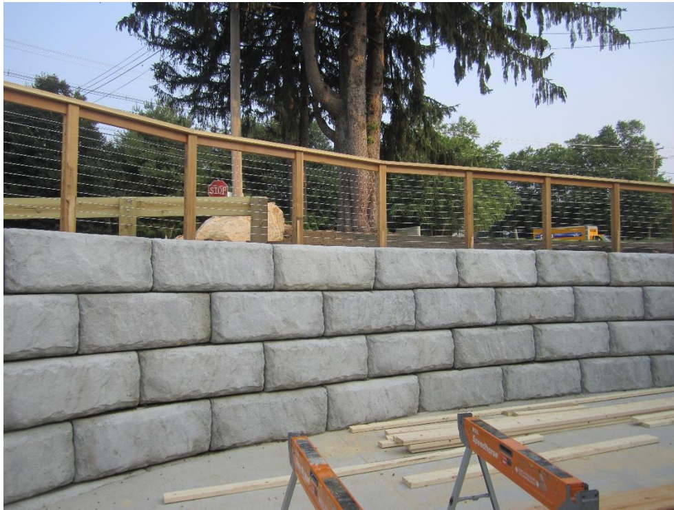
Retaining wall and fence in courtyard area
