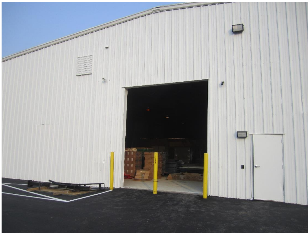
Bollards placed at loading area to building
