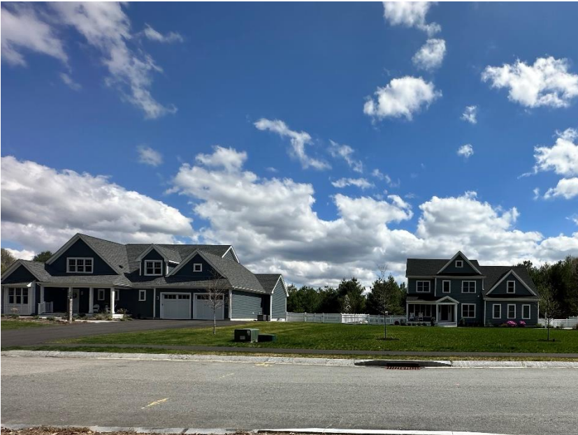
Photo 2: Completed houses, roadway, and lawn along Margaret's Cove, facing southeast.
