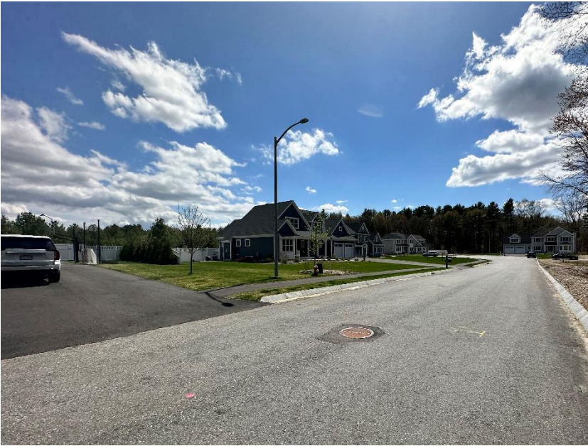
Photo 1: Completed houses, roadway, and lawn along Margaret's Cove, facing south.
