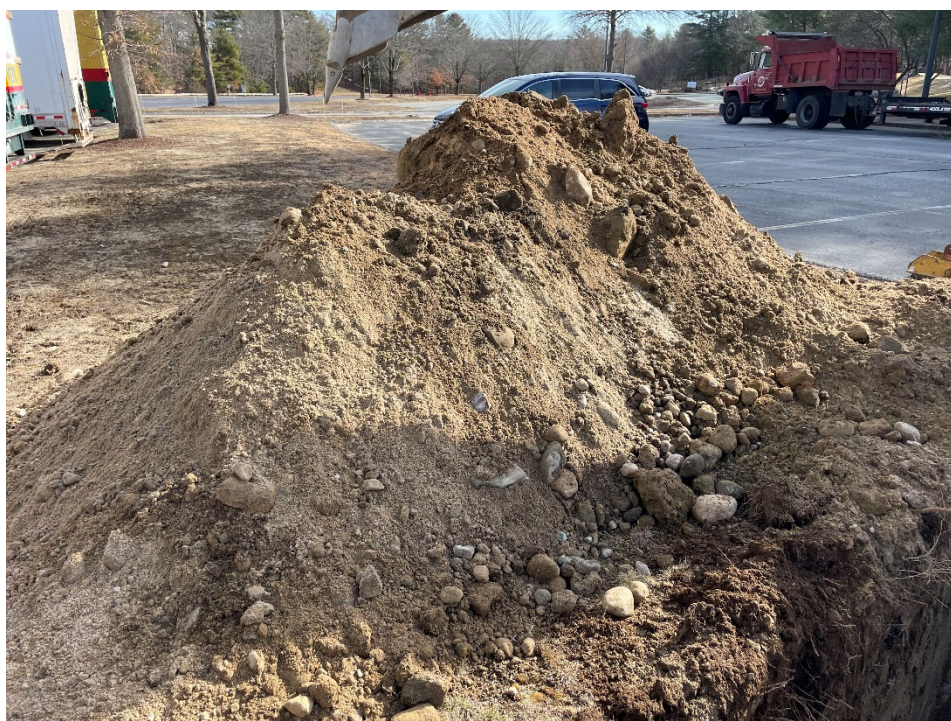
Photo #4: Looking northeast at soil excavated from test pit TP-2.
