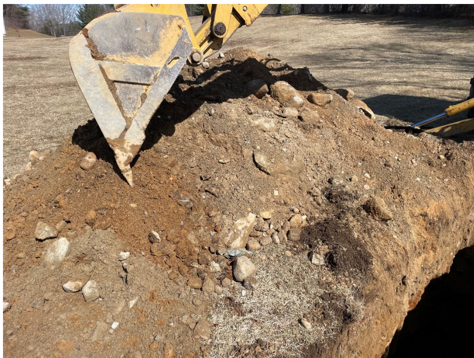
Photo #16: Looking northeast at soil excavated from test pit TP-8.
