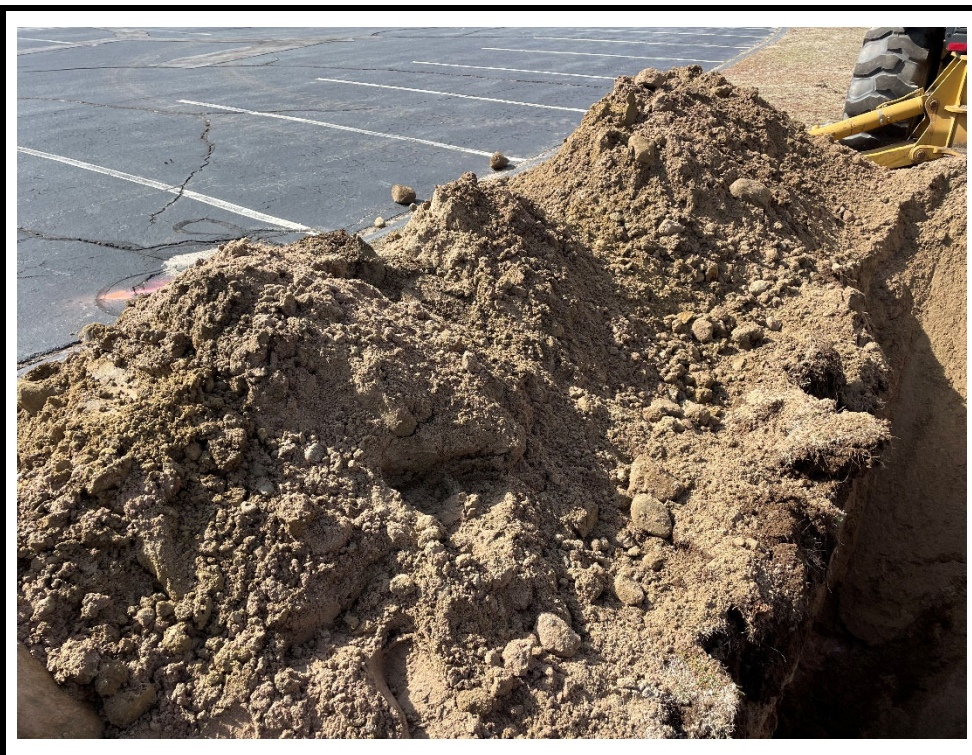
Photo #8: Looking southwest at soil excavated from test pit TP-4.
