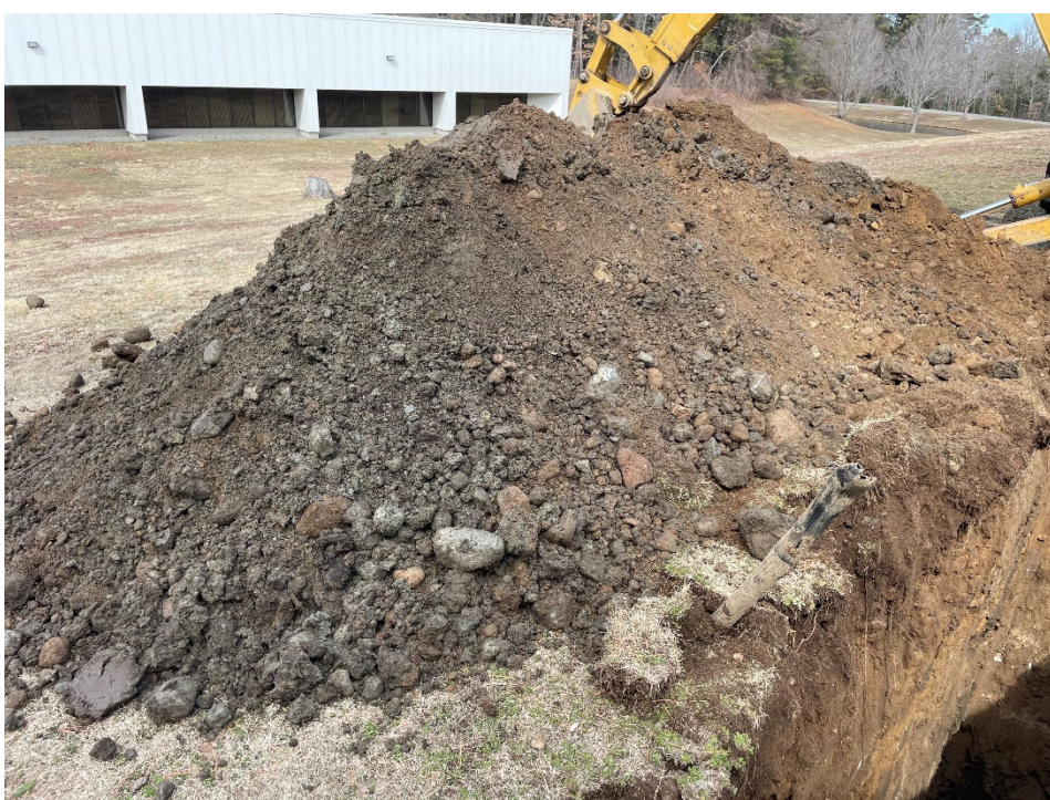
Photo #14: Looking north at soil excavated from test pit TP-7.
