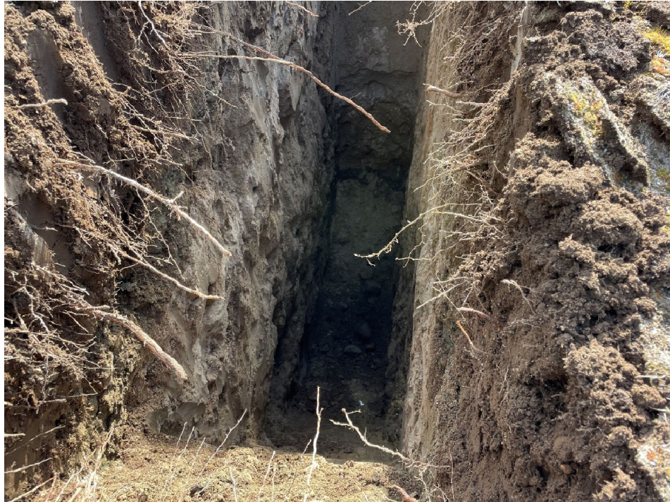
Photo #3: Looking southeast at test pit TP-2.
