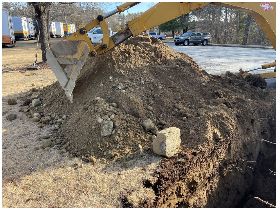
Photo #2: Looking northeast at soil excavated from test pit TP-1.
