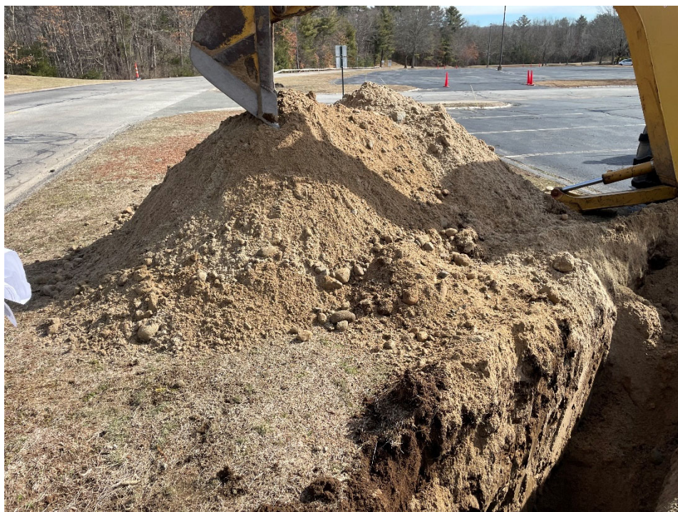
Photo #6: Looking northeast at soil excavated from test pit TP-3.
