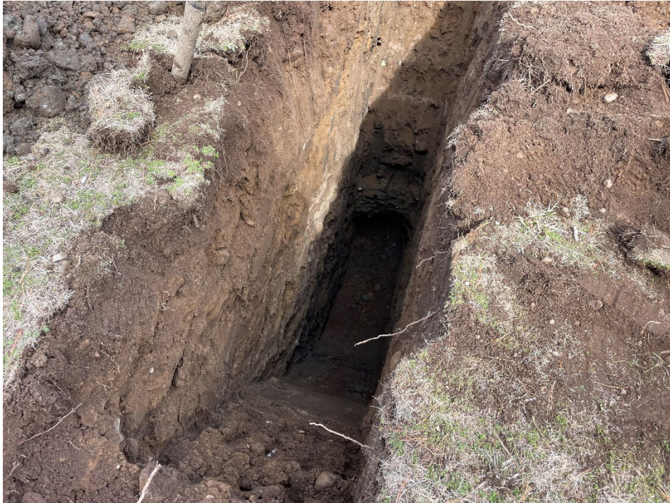
Photo #13: Looking northeast at test pit TP-7.
