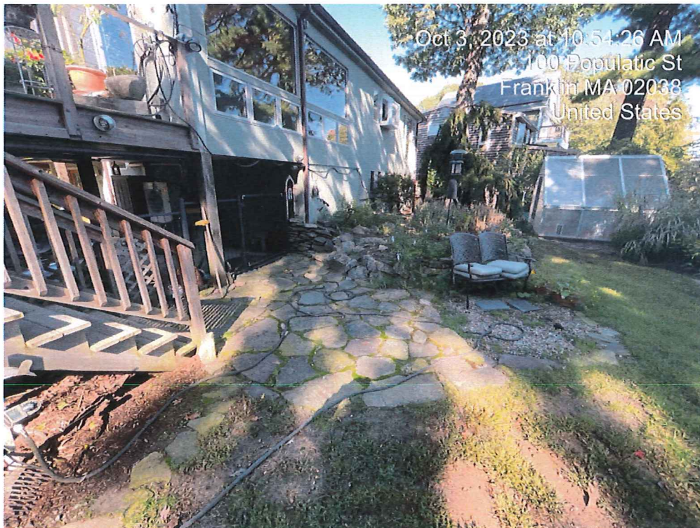
Figure 3: Existing patio area at rear of house.
