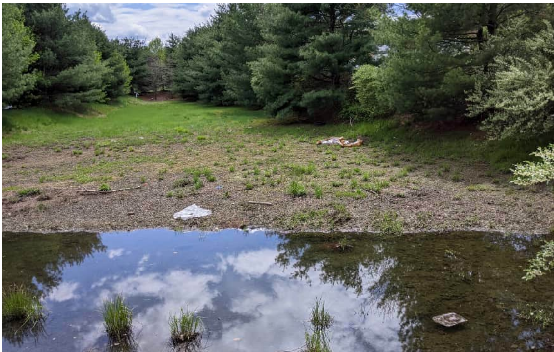
Typical view of a maintained stormwater basin at the northern end of the Site (157/161 Grove Street)—facing south.
