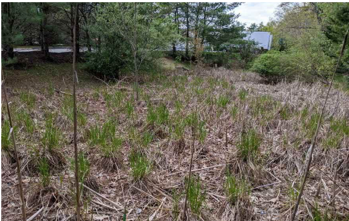
View of an unmaintained stormwater basin (WF11 Series IVW) at the northern end of the Site (157/161 Grove Street)—facing west.
