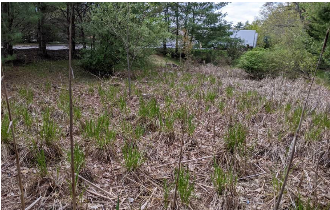
View of an unmaintained stormwater basin (WF11 Series IVW) at the northern end of the Site (157/161 Grove Street)—facing west.
