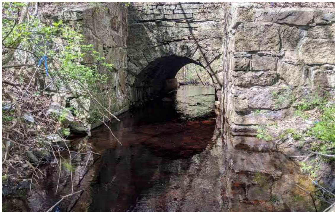
View of the culvert carrying Mine Brook, taken from the east side of Grove Street—facing west.
