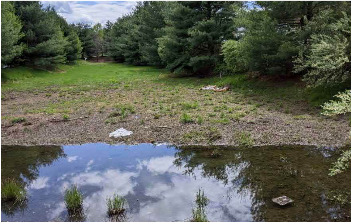
Typical view of a maintained stormwater basin at the northern end of the Site (157/161 Grove Street)—facing south.
