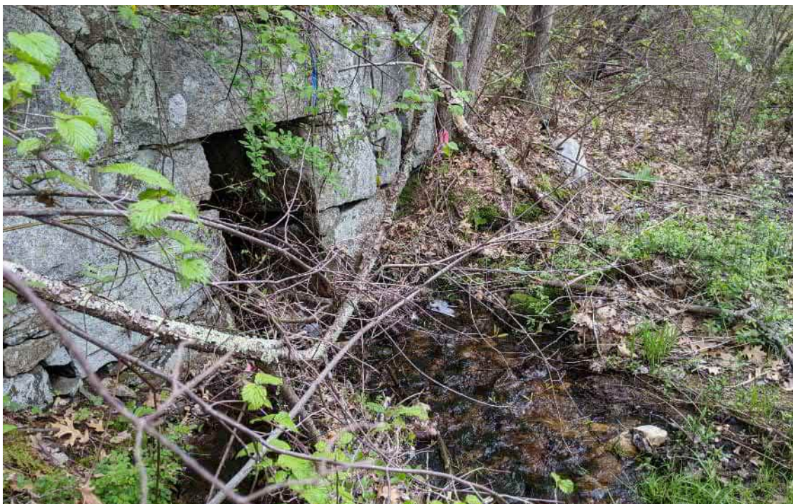
View of the unnamed tributary to Mine Brook flowing through a culvert under the Southern New England Trunkline Trail—facing northeast.
