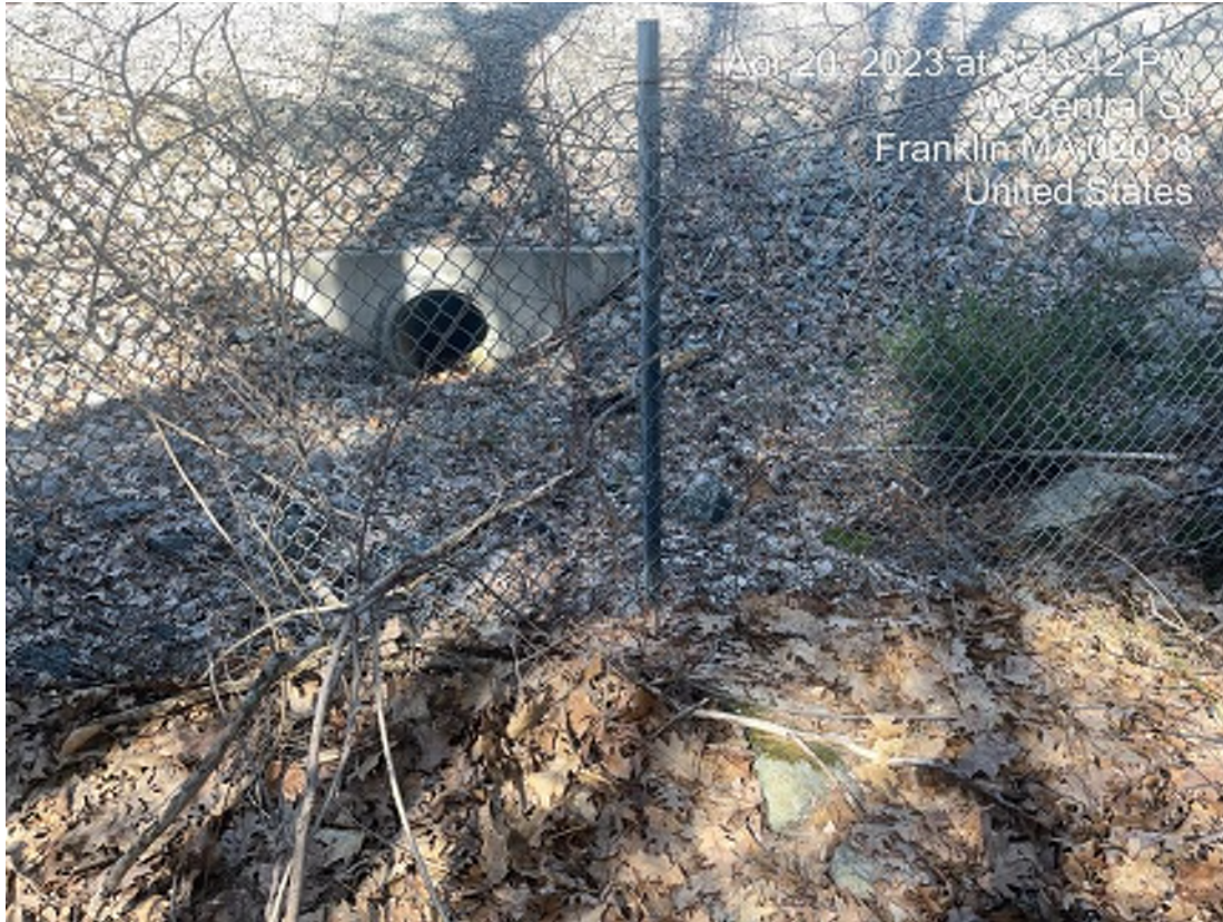
Photo 4. Photo of culvert at downgradient terminus of BMP on site.
