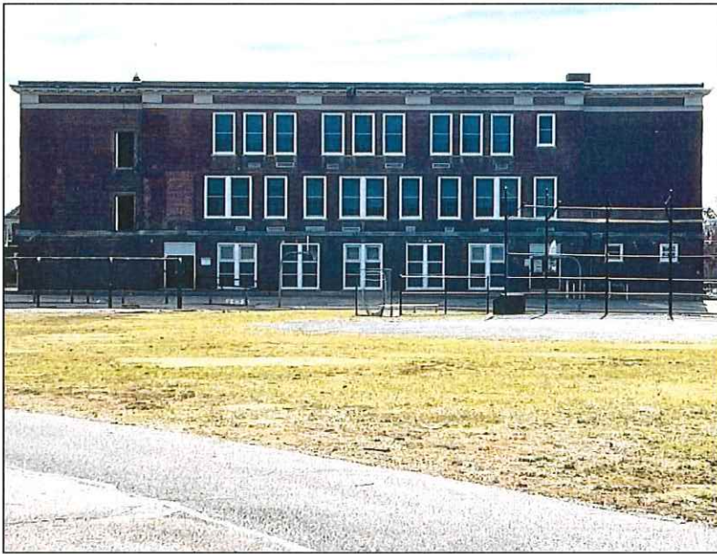
North side of building, with playground and ballfield.
