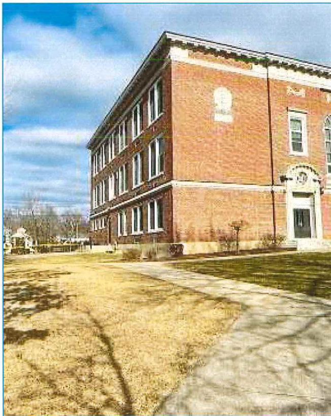
Southwest corner of building.
