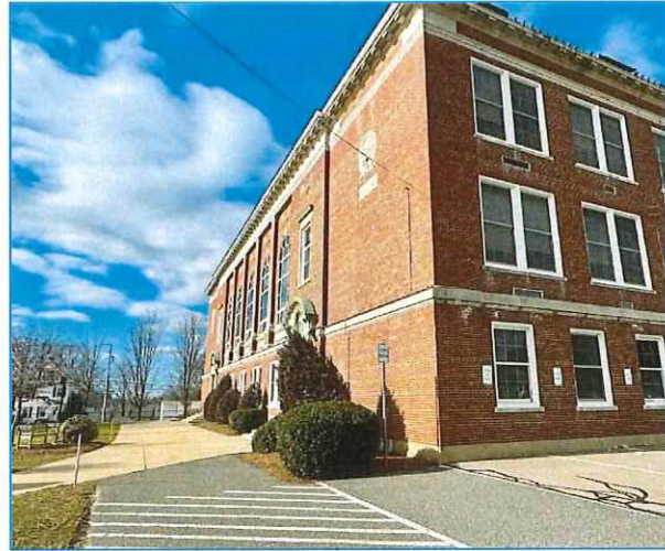
Southeast corner of building.
