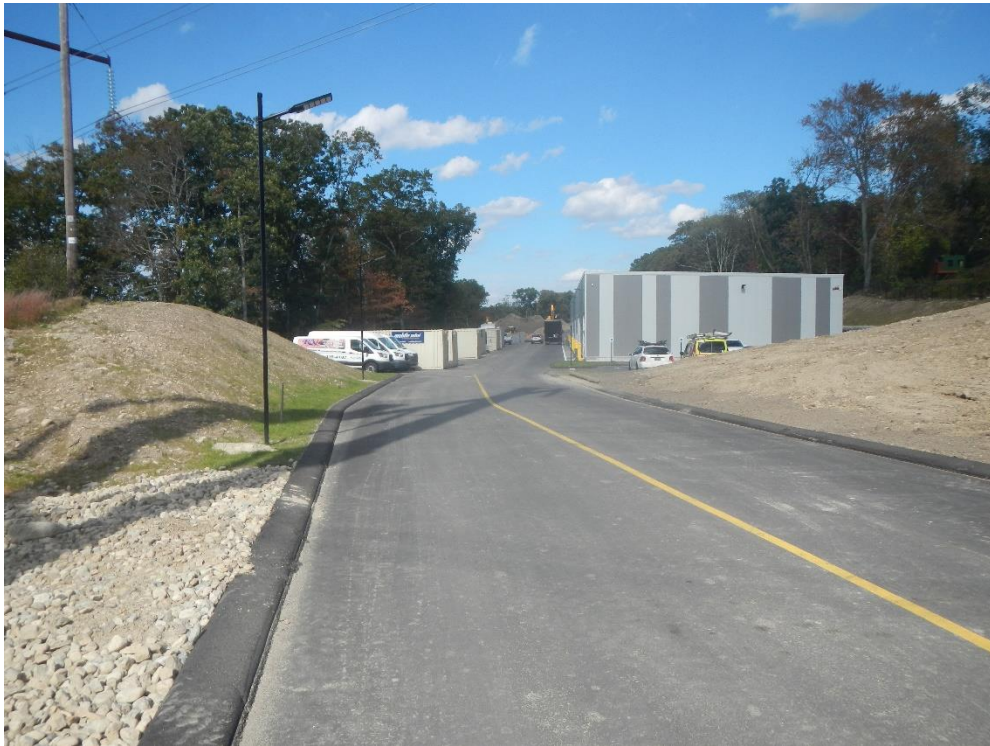
Site driveway facing north, showing typical lighting, storage containers, and easement access (left)
