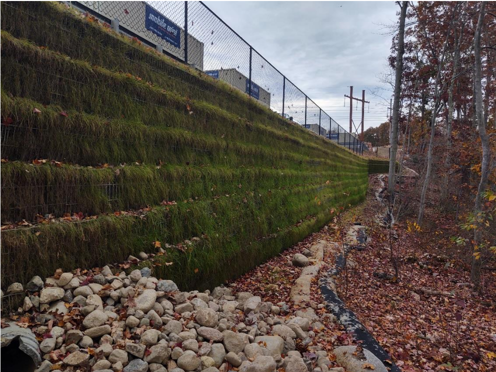
Westerly retaining wall
