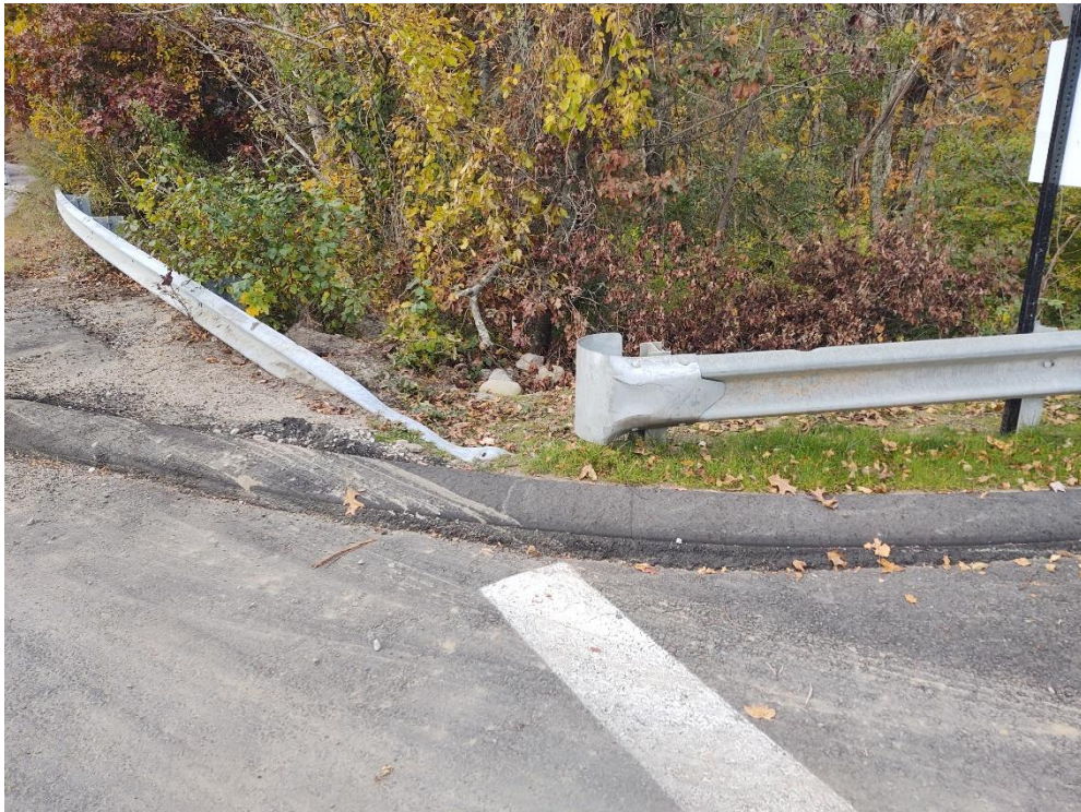
Guardrail with terminal end section installed
