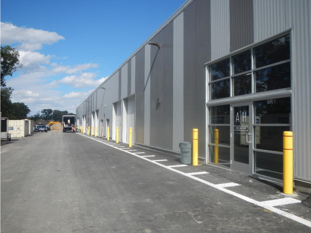
Typical face of building showing wall mounted lighting and bollards
