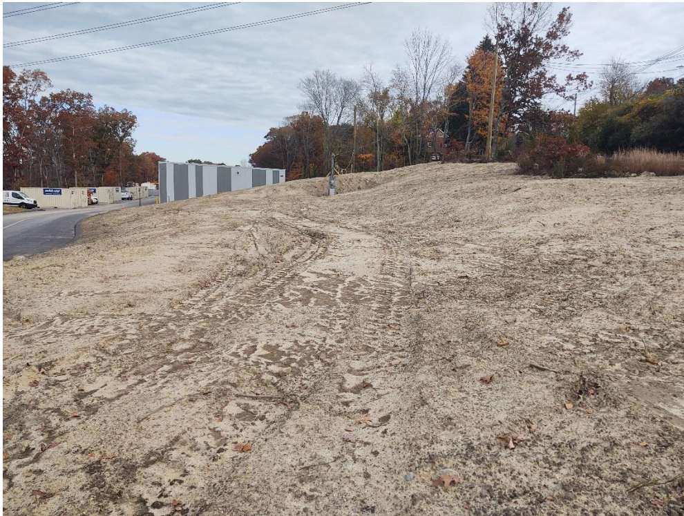
Slope recently hydroseeded
