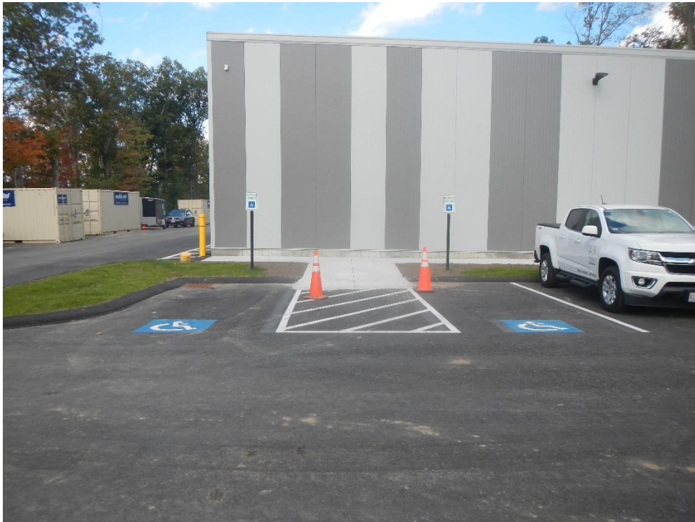
Accessible parking area and ramp
