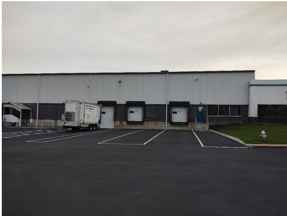
Completed loading dock area
