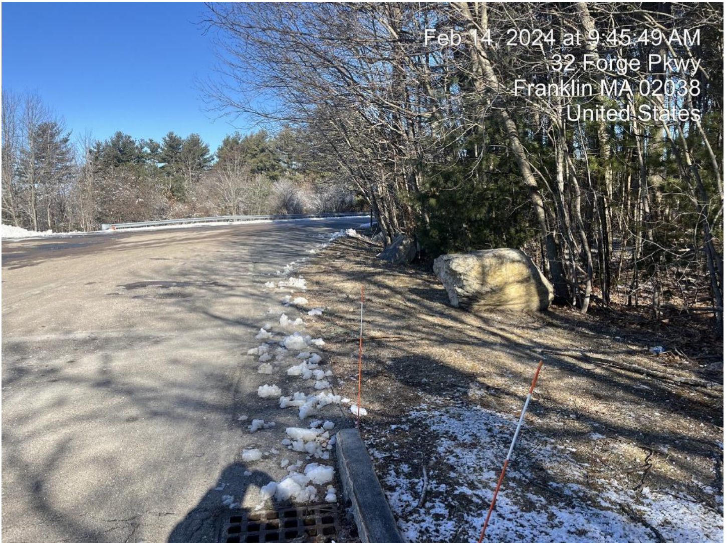
Figure 5: Approximate location of easternmost utility pole to be embedded within mowed right of way
