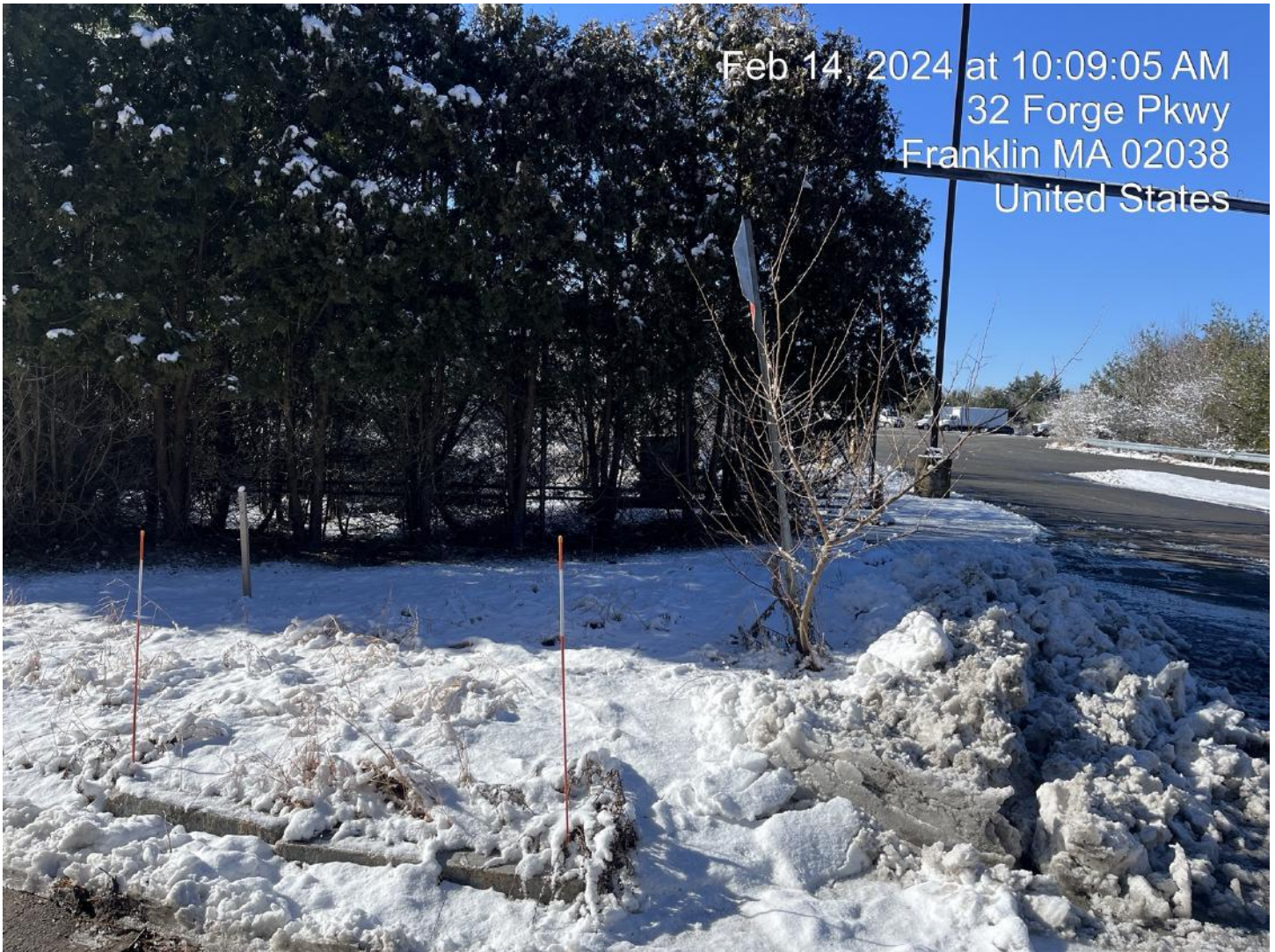
Figure 6: Approximate location of second utility pole to be embedded within mowed right of way between access roads. Wooden stake demarcates location of proposed pole.
