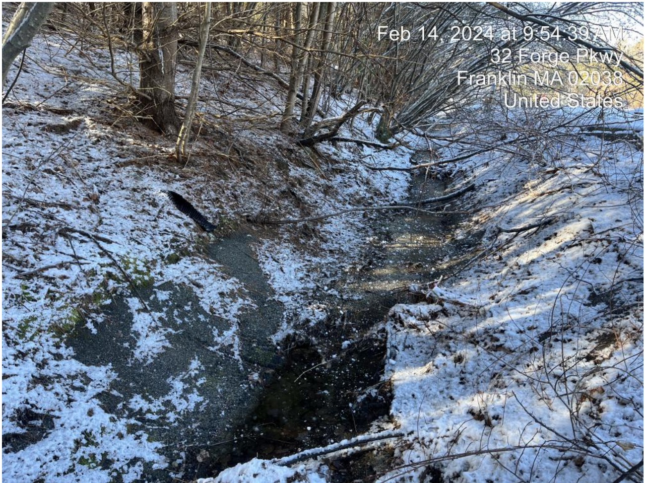
Photo 2. Concrete lined swale delivering stormwater adjacent to parking lot.
