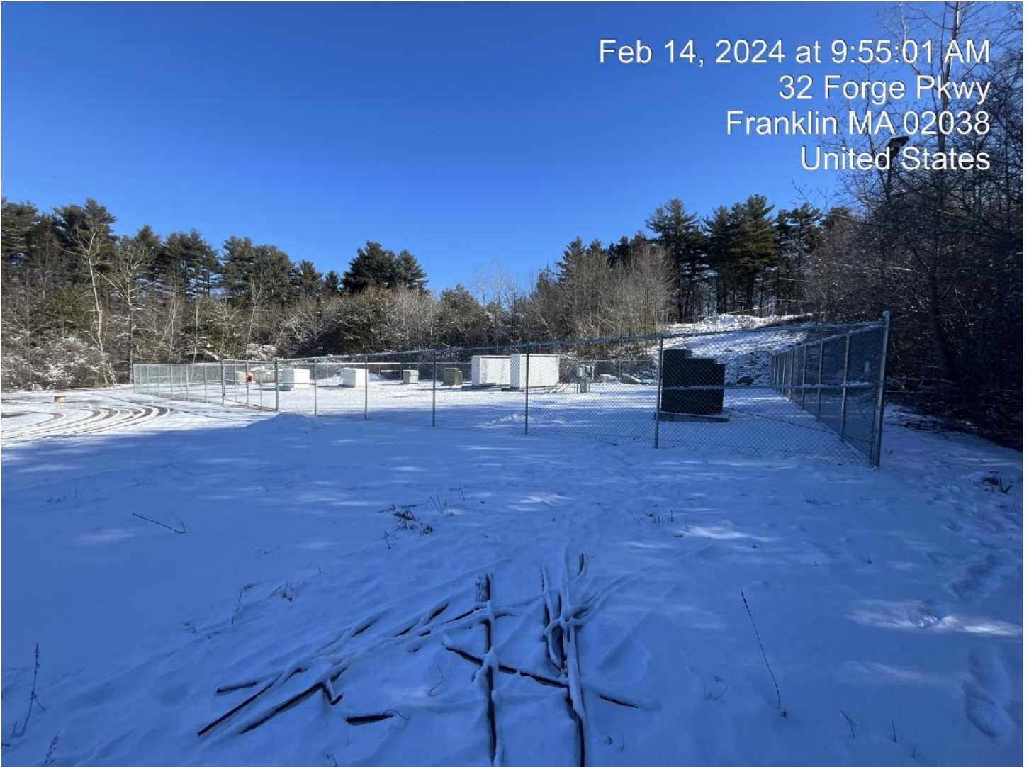
Figure 2: Existing generator pad within parking lot.
