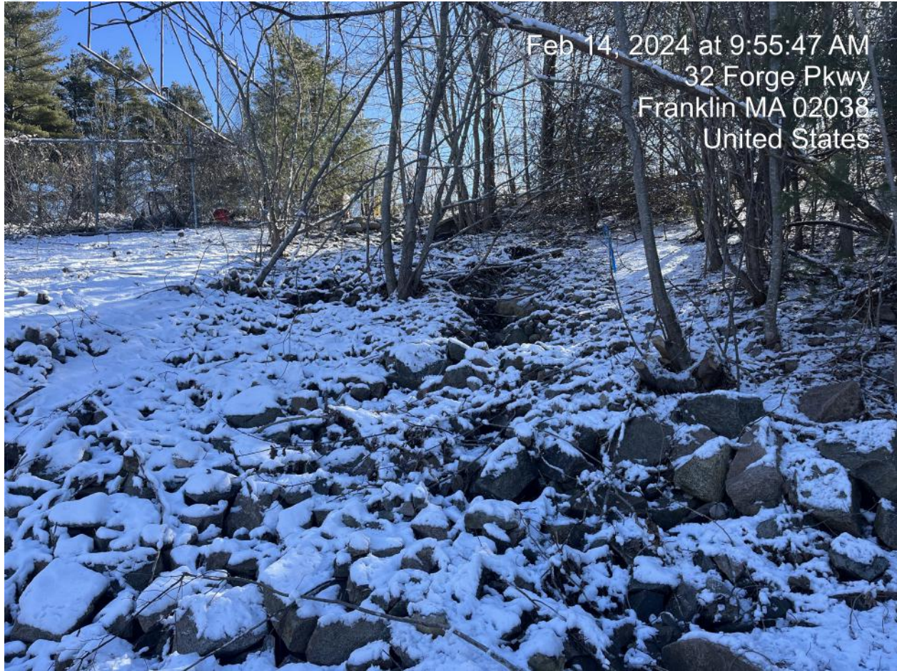
Photo 3. Rip-Rap drainage swale taking stormwater under site access drive
