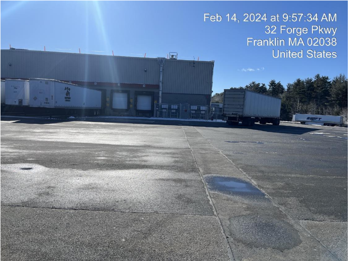
Figure 1: View of existing warehouse. Solar transformers can be seen against building.
