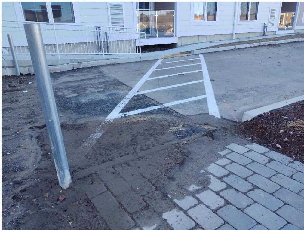
Walkway that is anticipated to require detectable warning.
