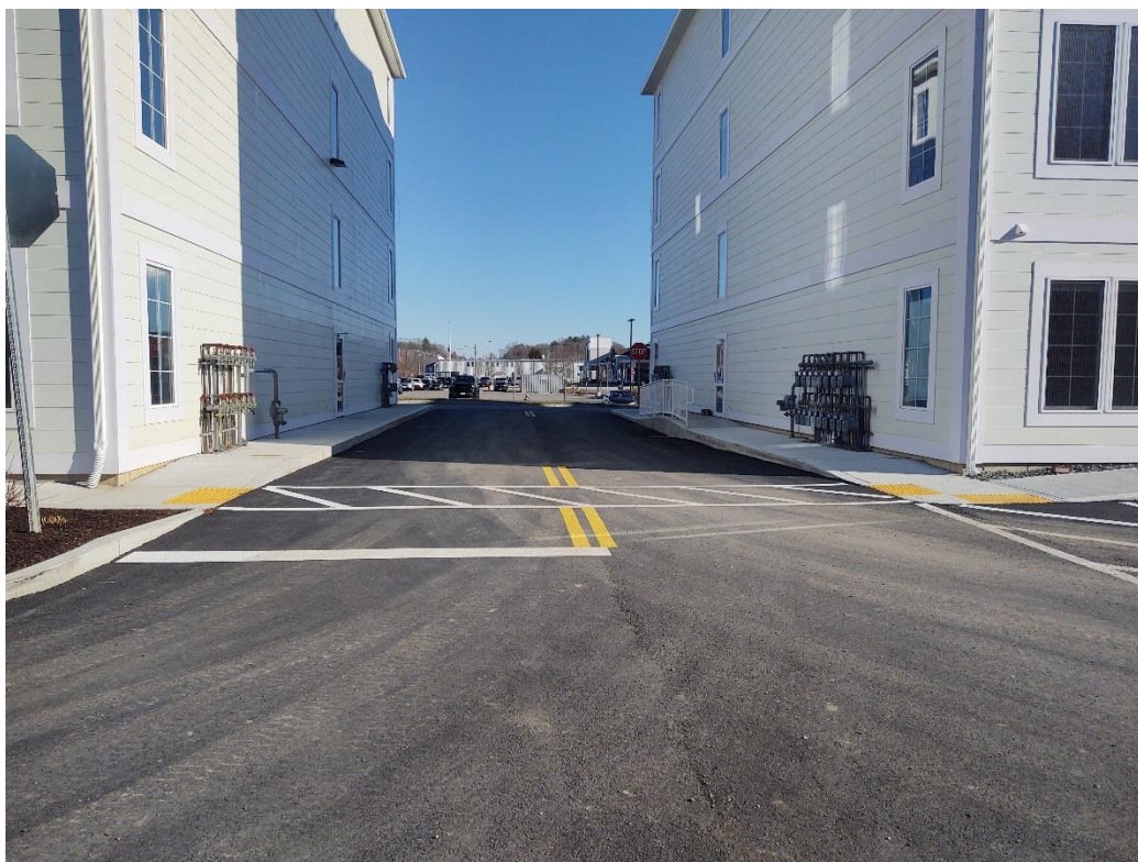
Access drive between Buildings A and B
