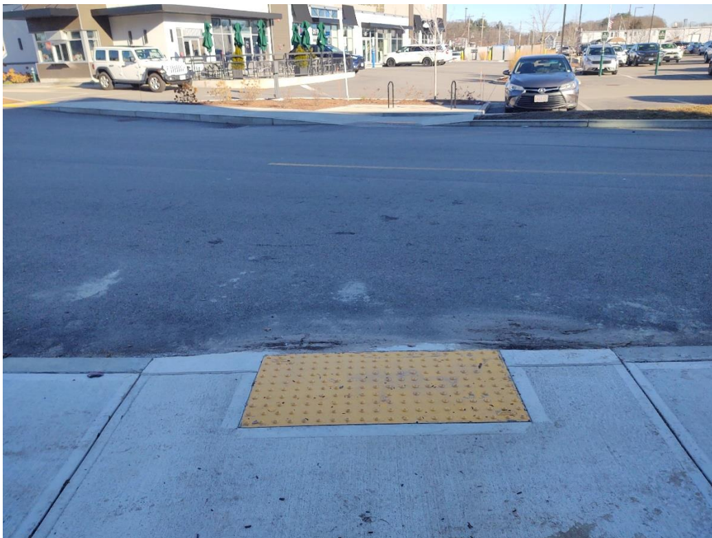
Unstriped crosswalk from Building B to Building C
