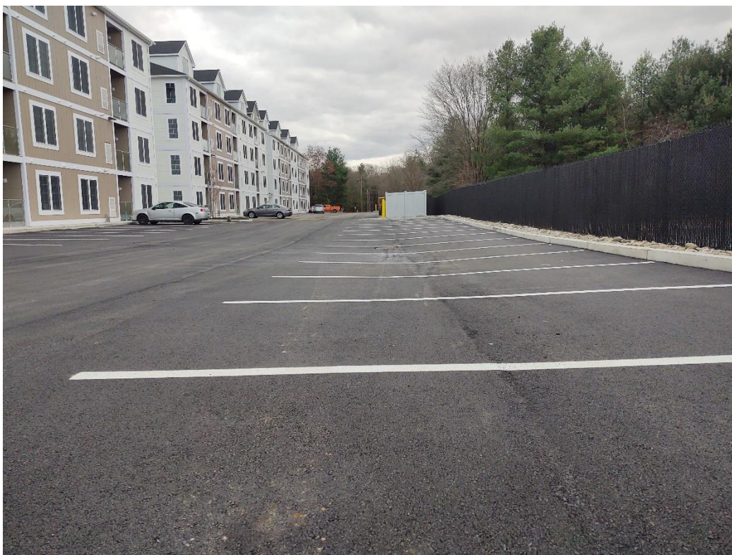
Typical parking area
