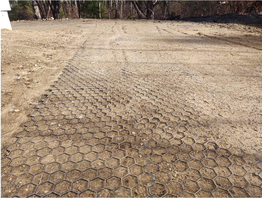
Geogrid fire access lane
