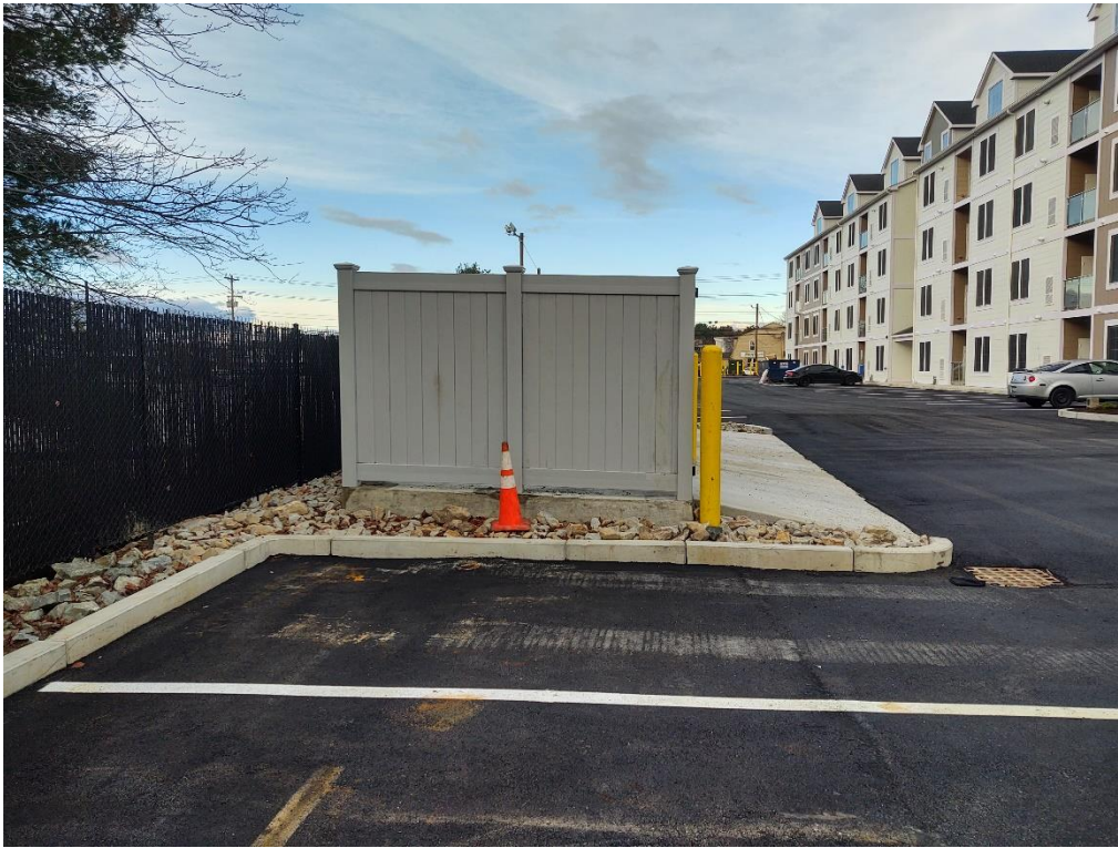
Dumpster pad with steep ramp access
