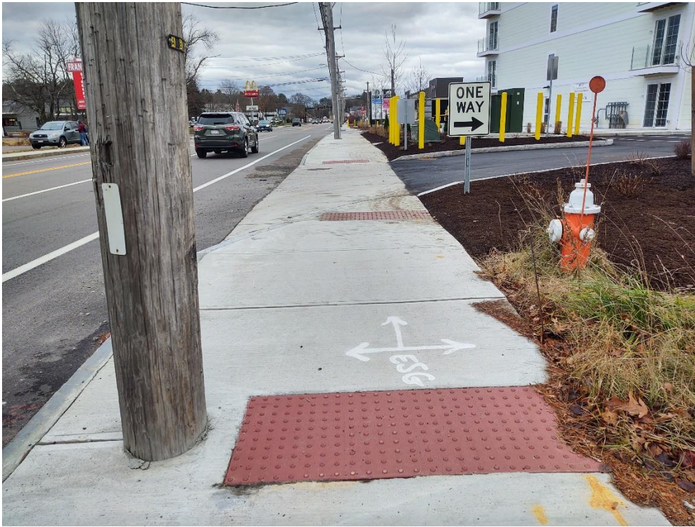
Continuous concrete walk across westerly driveway
