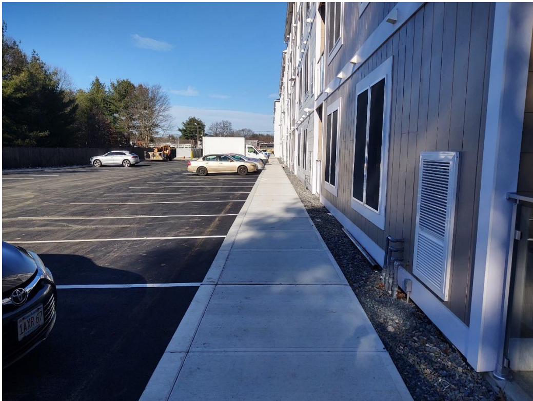
Typical sidewalk along Building B
