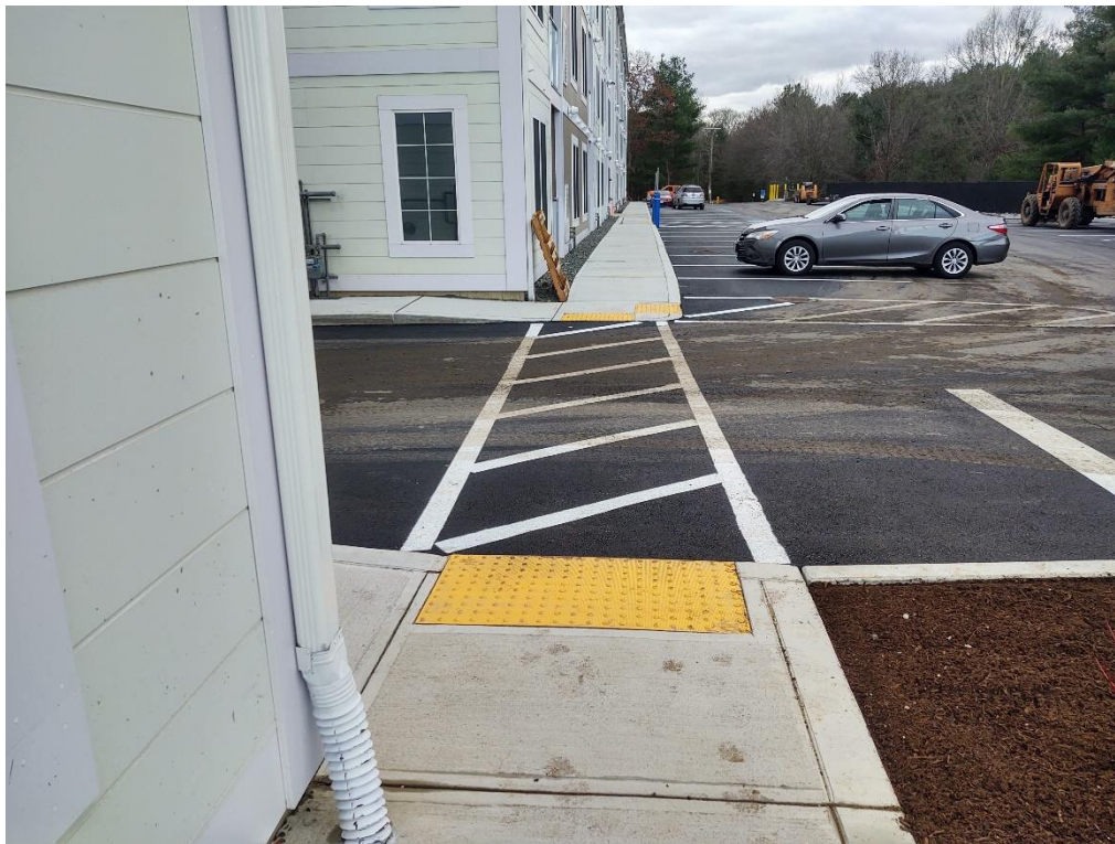
Accessible route between Buildings A and B
