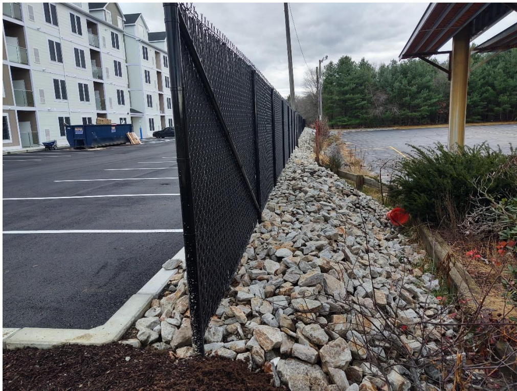
Typical screening fence with rip rap slope behind
