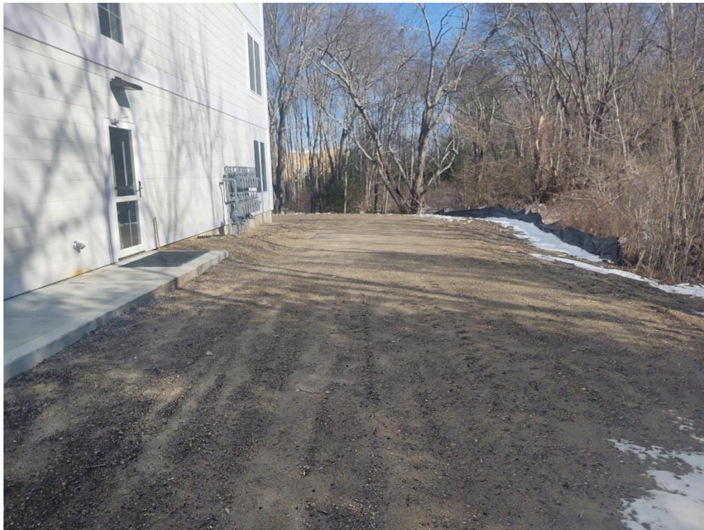
Completed geogrid fire access lane – seed to germinate in spring
