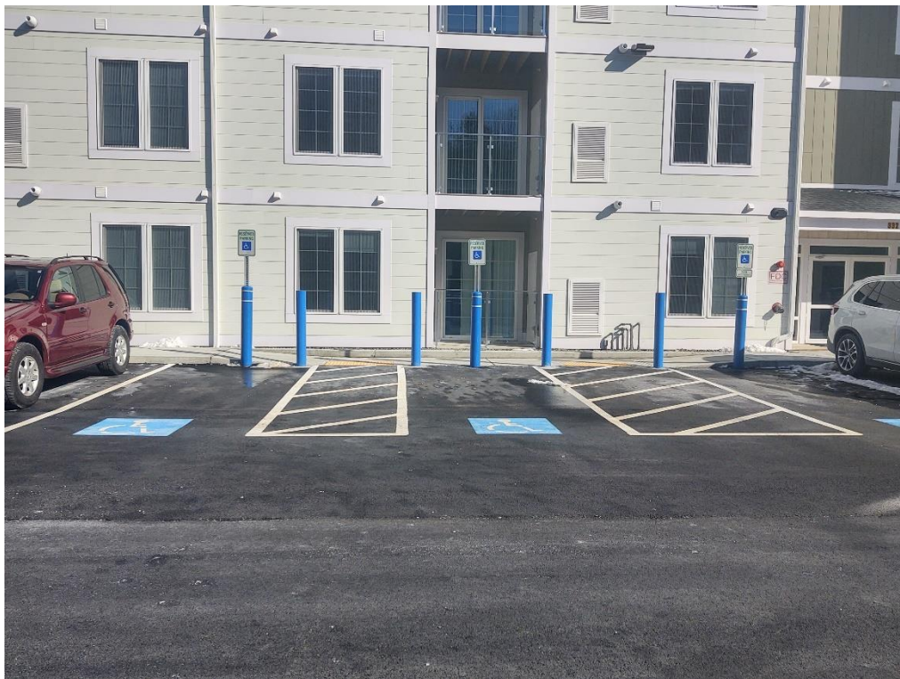
Accessible parking with bollards to prevent vehicle encroachment onto sidewalk
