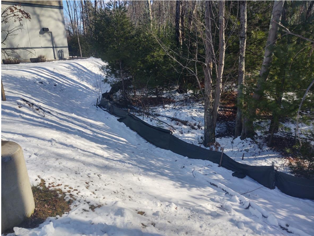
Silt fence that requires removal in coordination with Conservation Agent
