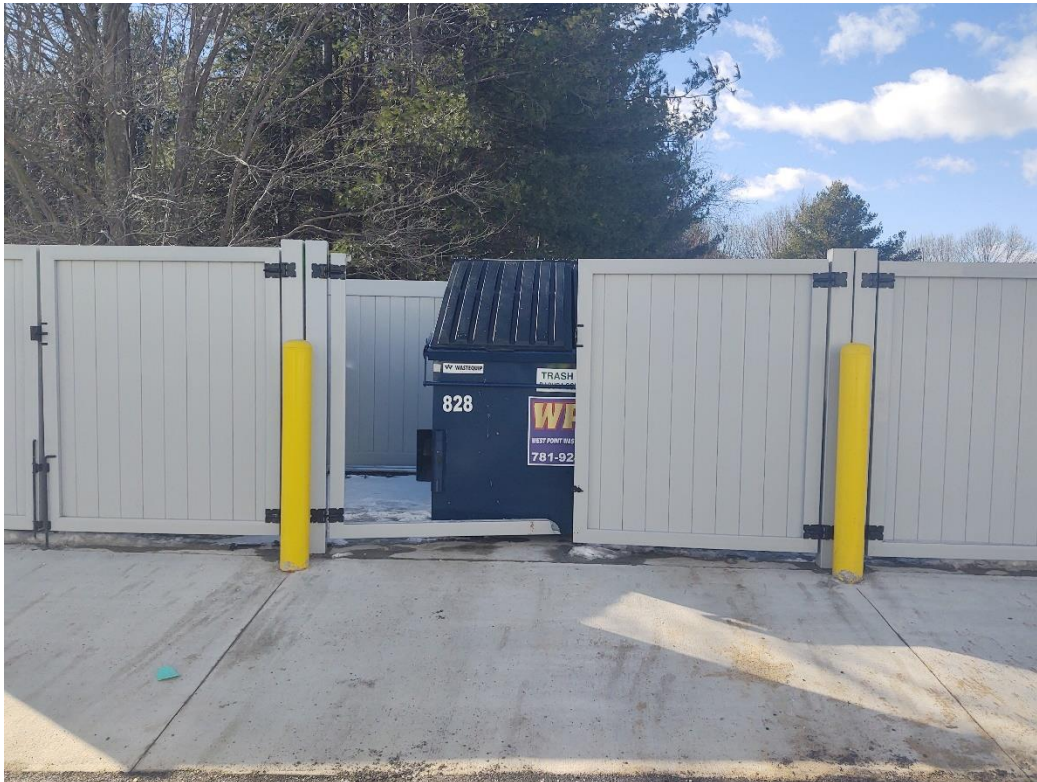
Dumpster enclosure currently being repaired
