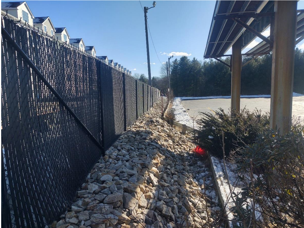
Completed rip rap slope
