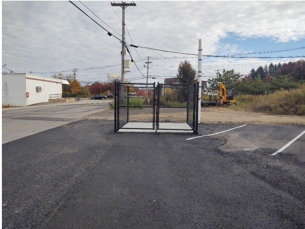
Dumpster enclosure and pole for signage
