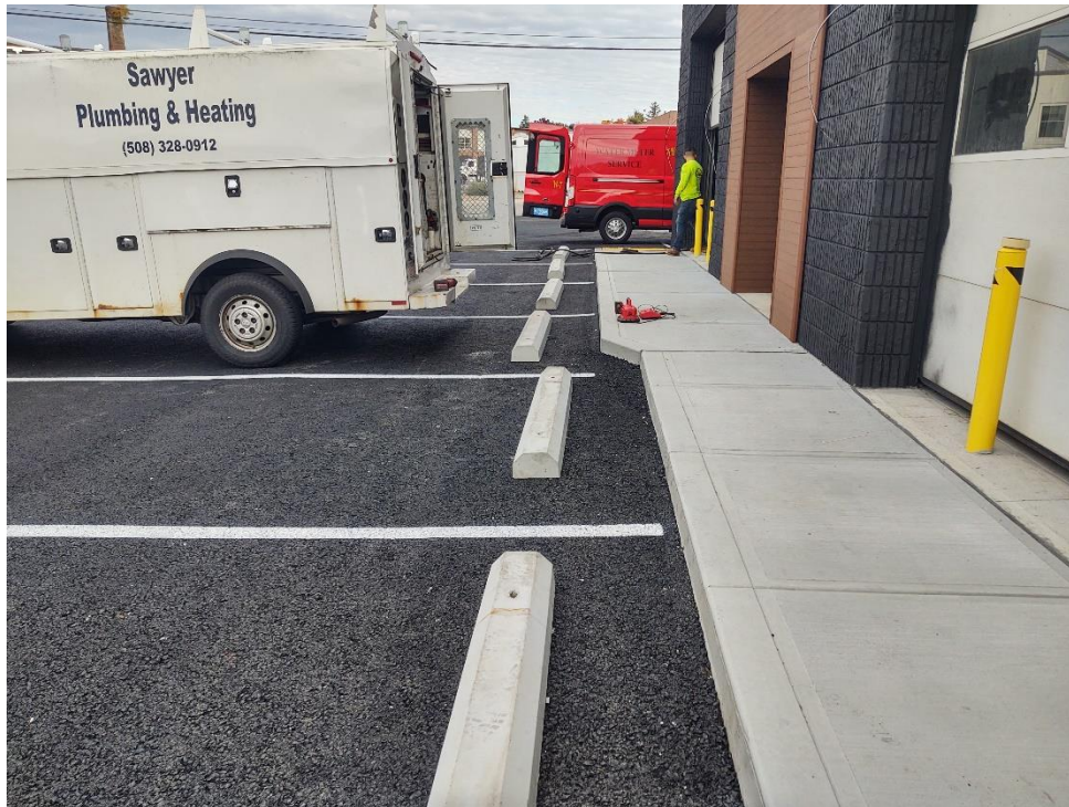
Parking adjacent to building. Bollards installed at all overhead doors.
