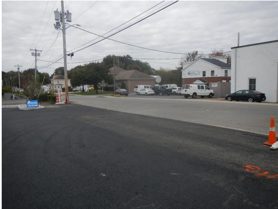
Typical pavement match to Cottage Street
