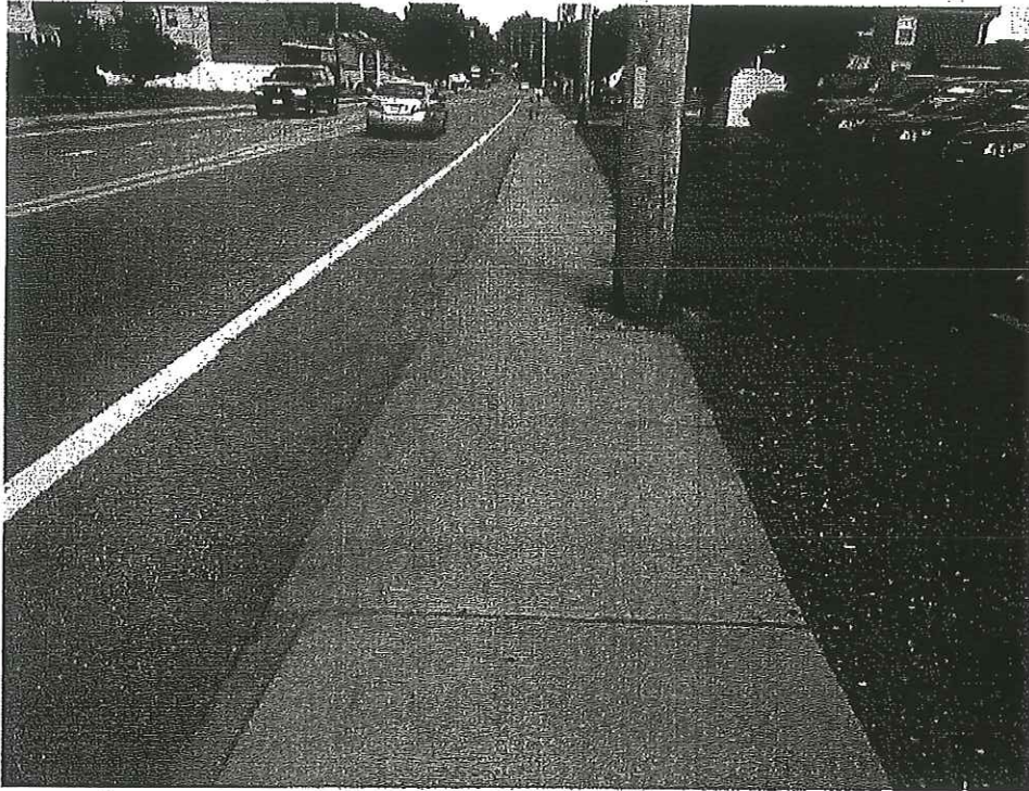
Abandoned curb cut remains
