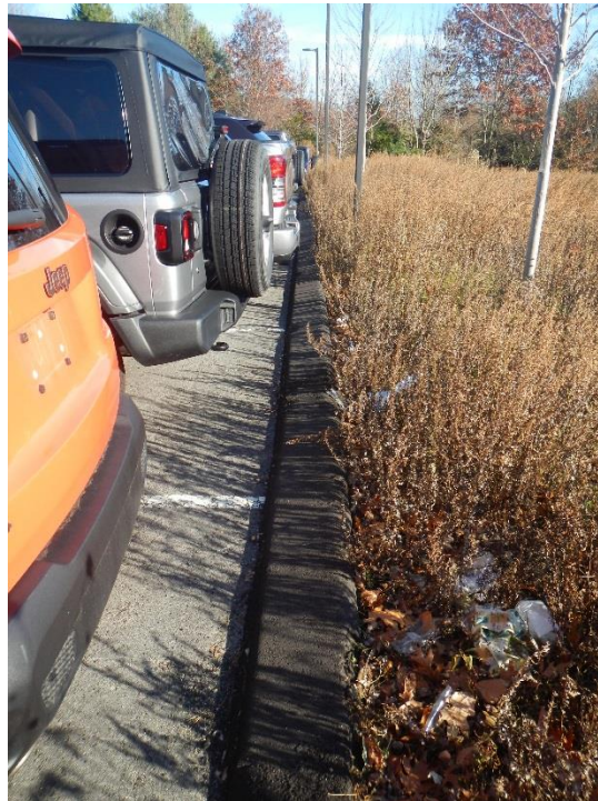
Typical repair to bituminous curbing
