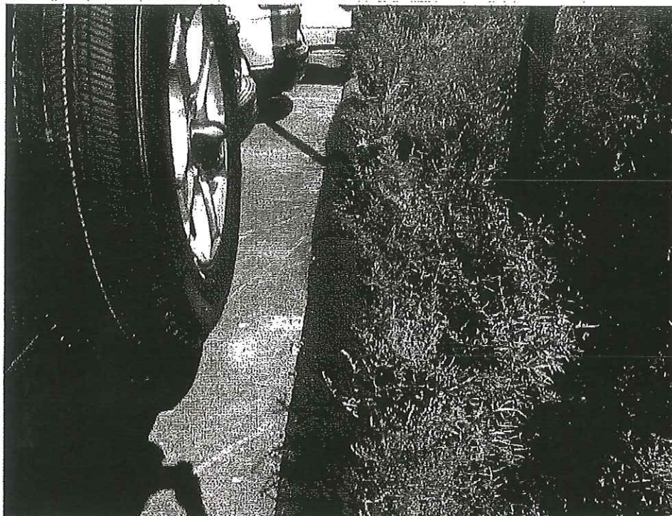
Typical bituminous curbing repaired
