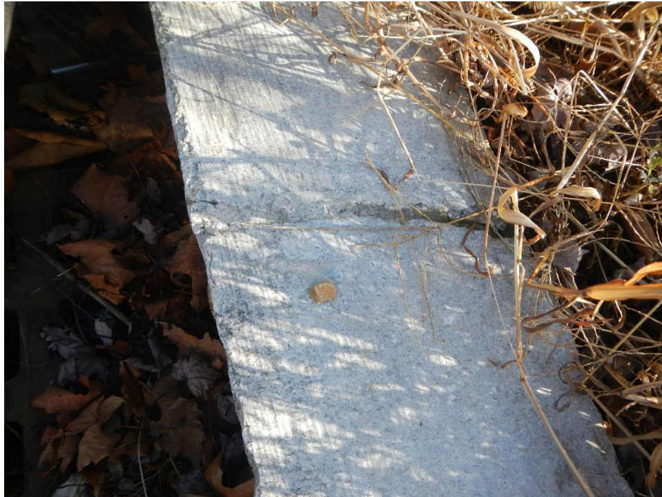
Repaired granite inlet stone
