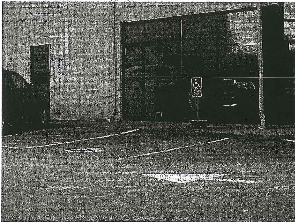
Installed handicap signage
