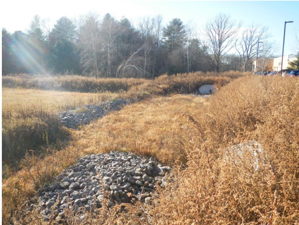
Typical stormwater basin in good working order
