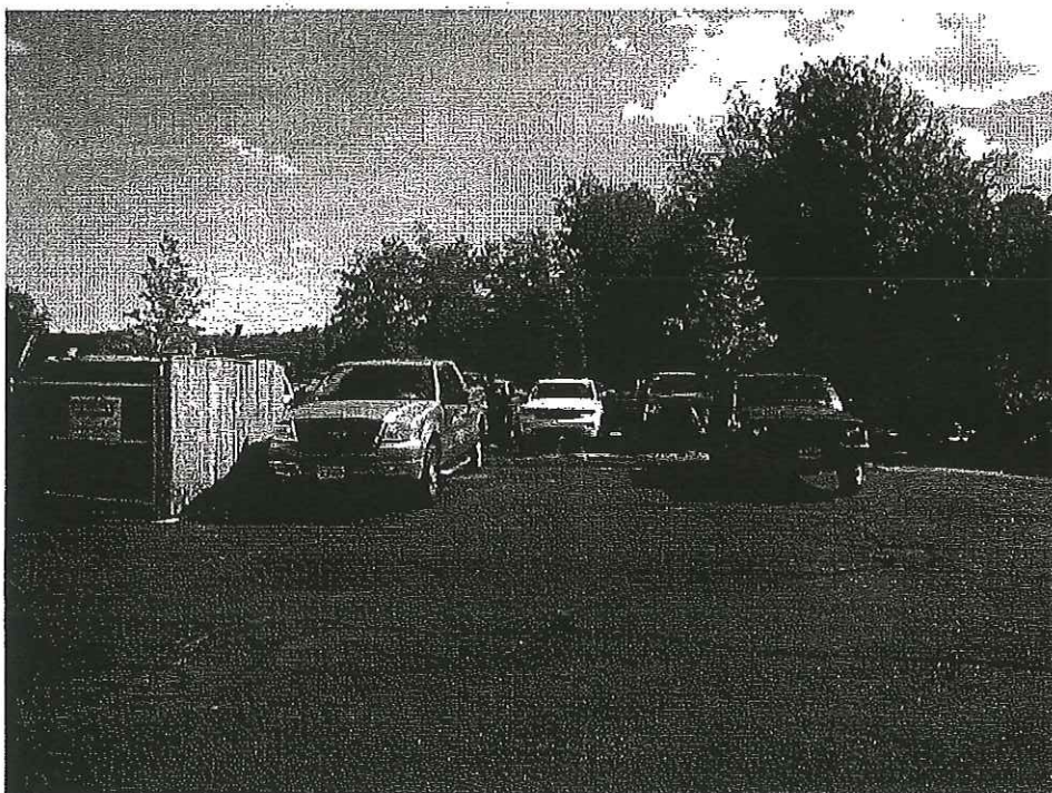
Four unstriped parking spaces adjacent to dumpster
