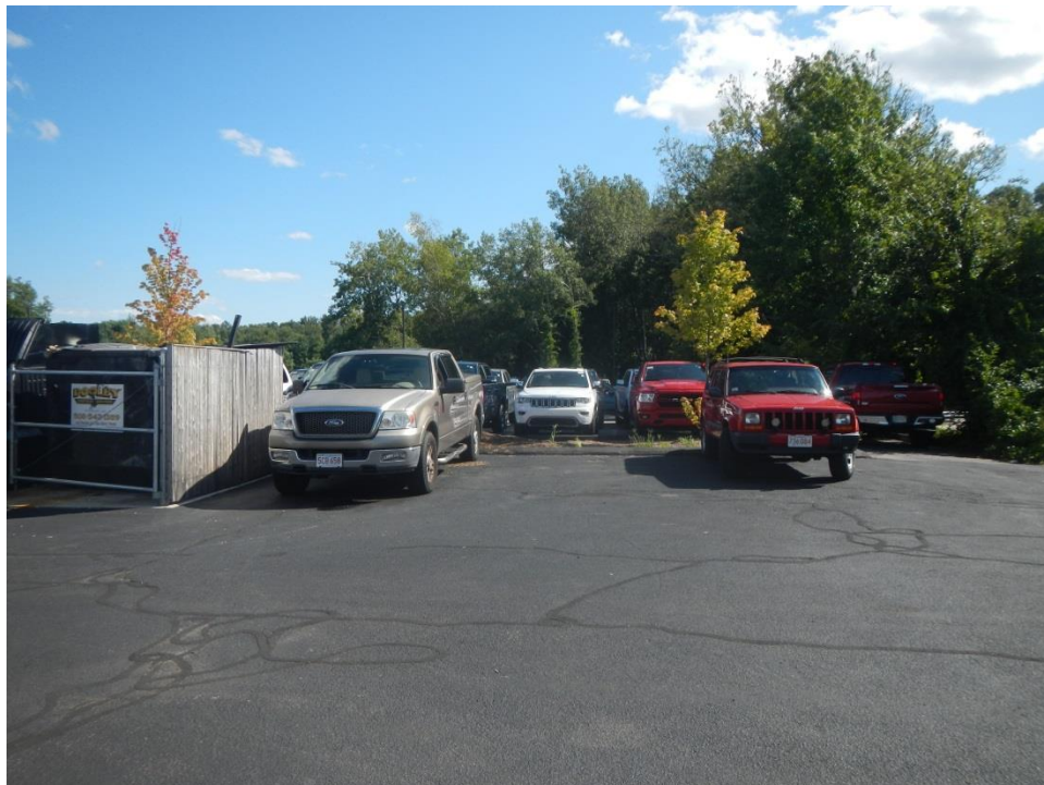
Four unstriped parking spaces adjacent to dumpster (August 2018)
