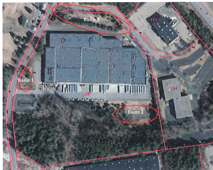
Photo 1. Red highlighted areas of concern; basin to the north, south and front of the building
