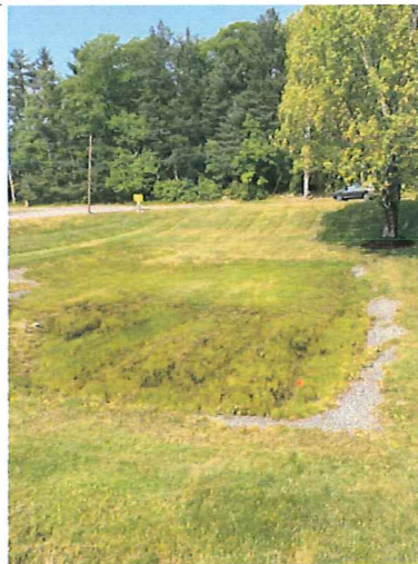
Photo 3. Basin 1., looking west; observing all of the detention basin except the culvert shown in the other photo. Culvert is located to the left of this photo.
