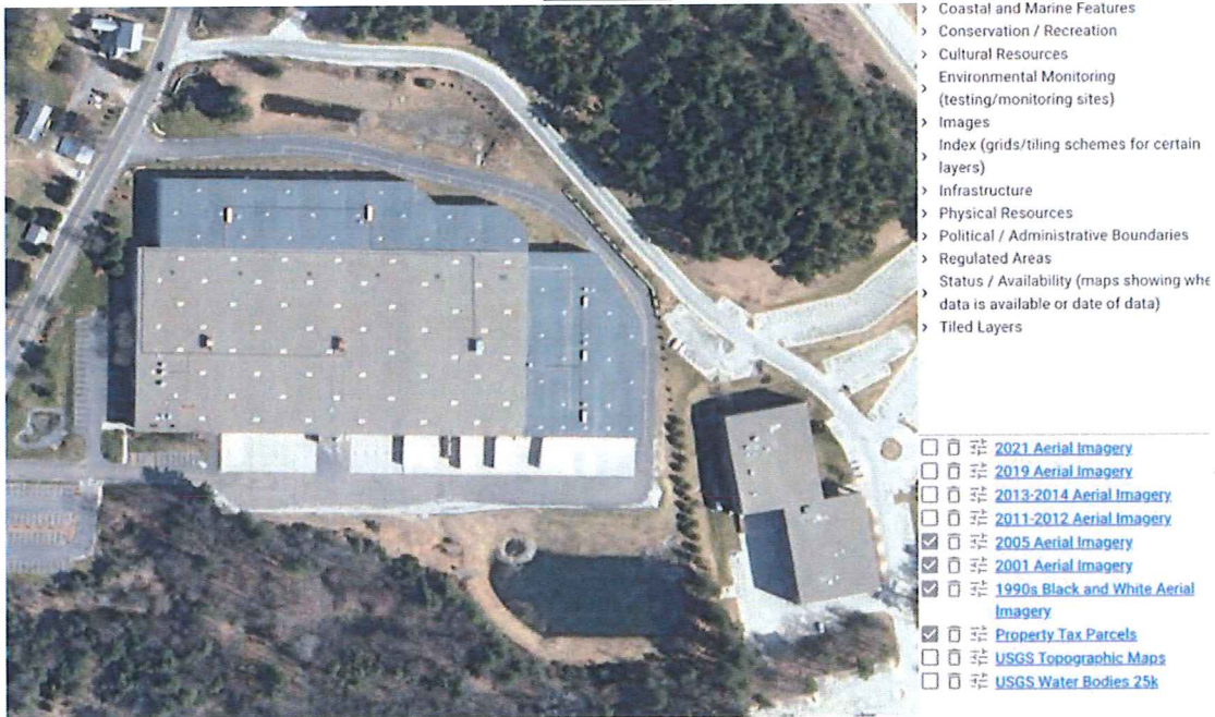
MassMapper aerial imagery from 2005 showing additional parking lot space (southwest of the building). Notice both detention basins filled with water and functional.
