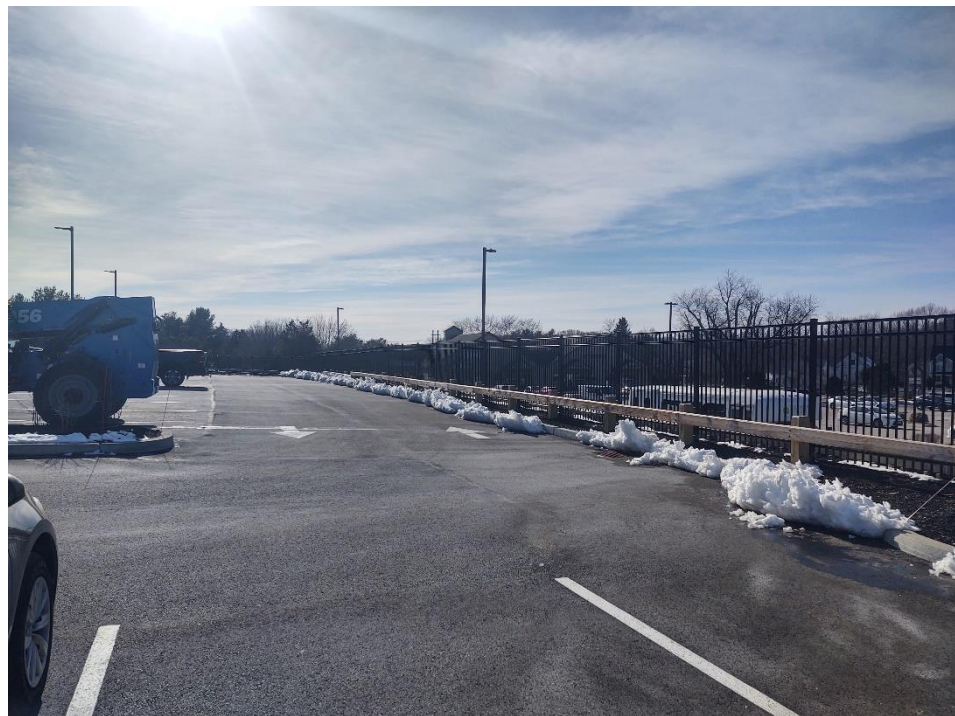
Typical ornamental fence and wooden guardrail
