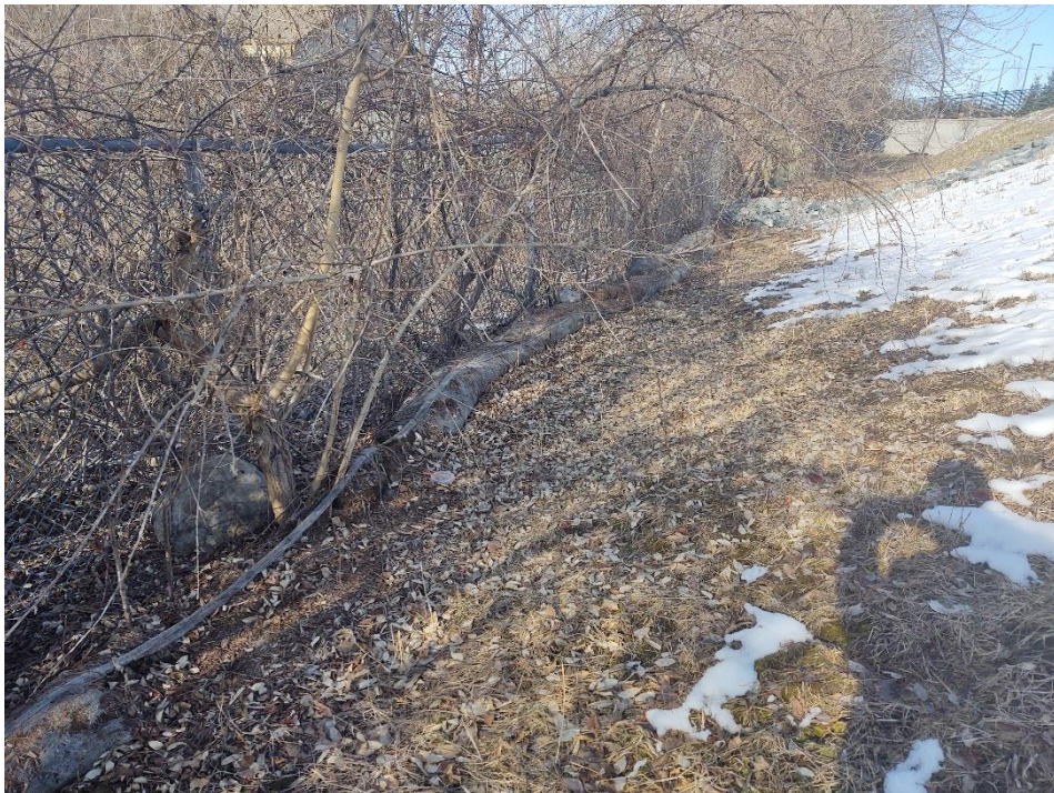
Remnant erosion controls that should be removed in coordination with Conservation Agent
