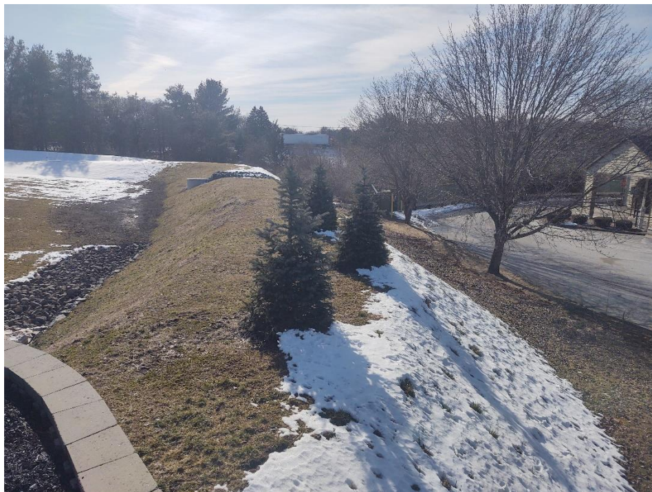
Spruce trees relocated to top of basin berm
