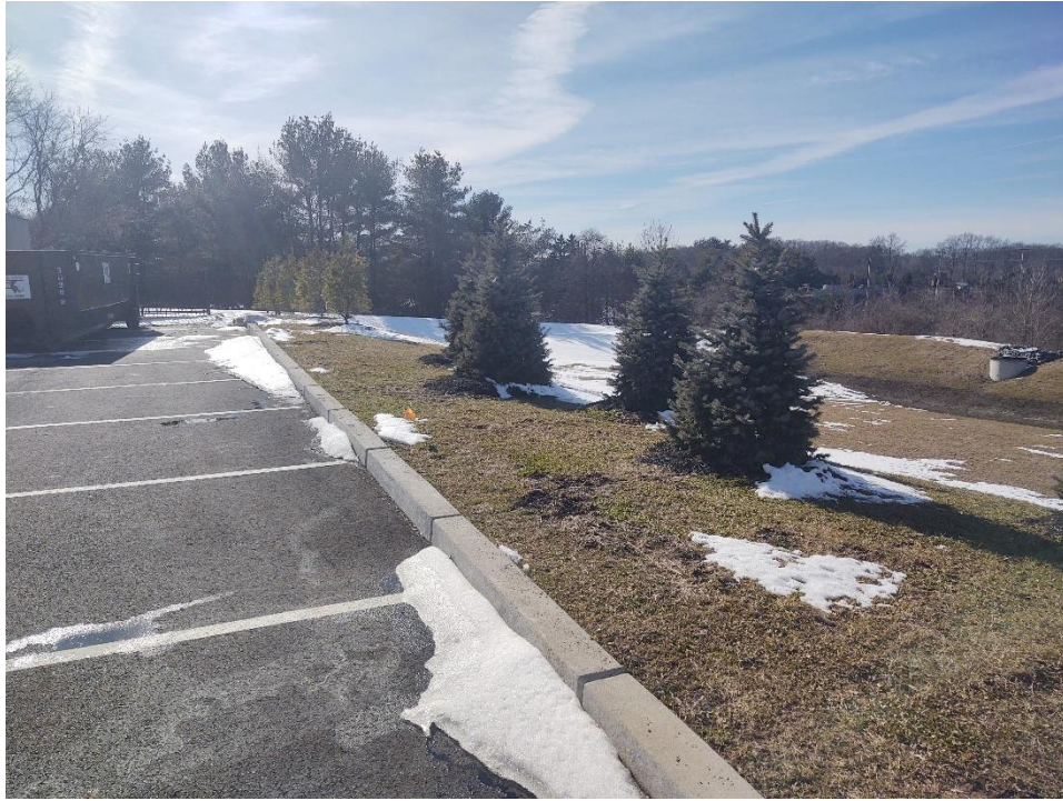
Typical plantings adjacent to infiltration basin
