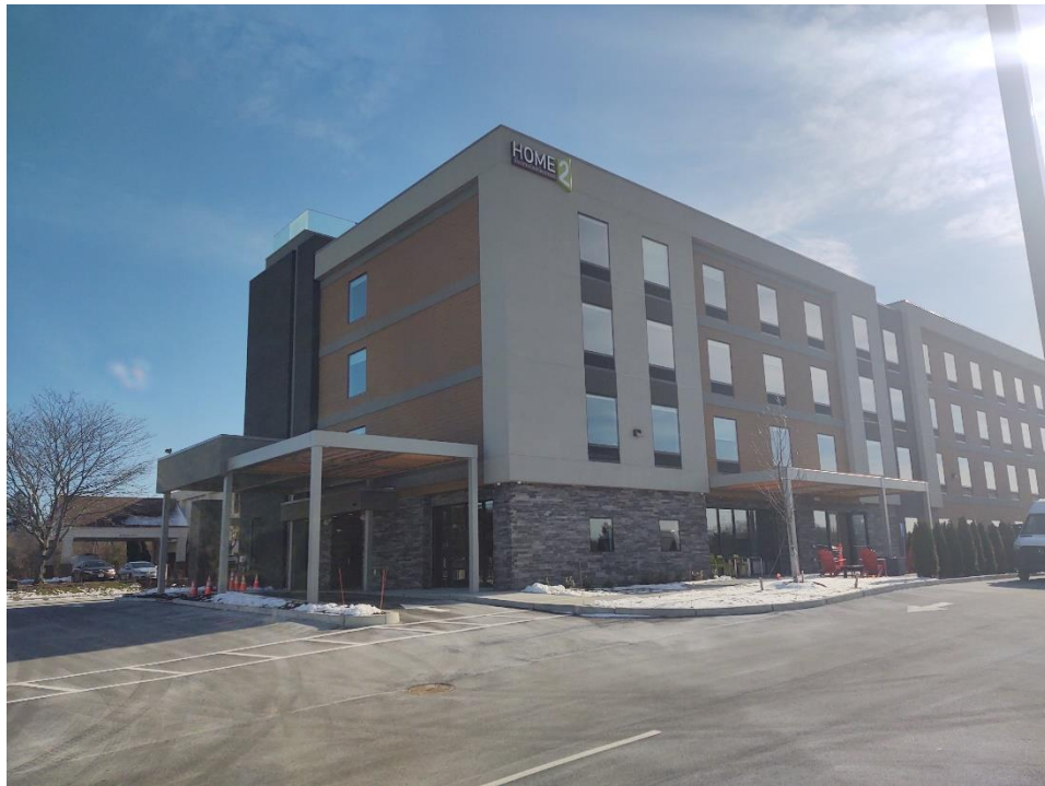
Building view from Union Street
