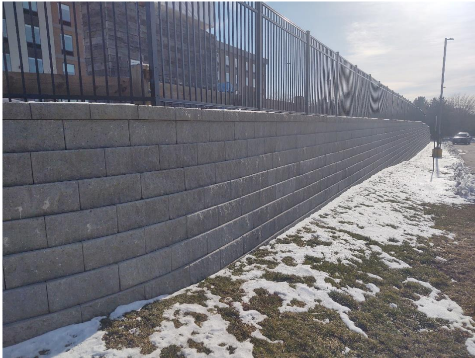
Retaining wall along westerly property line
