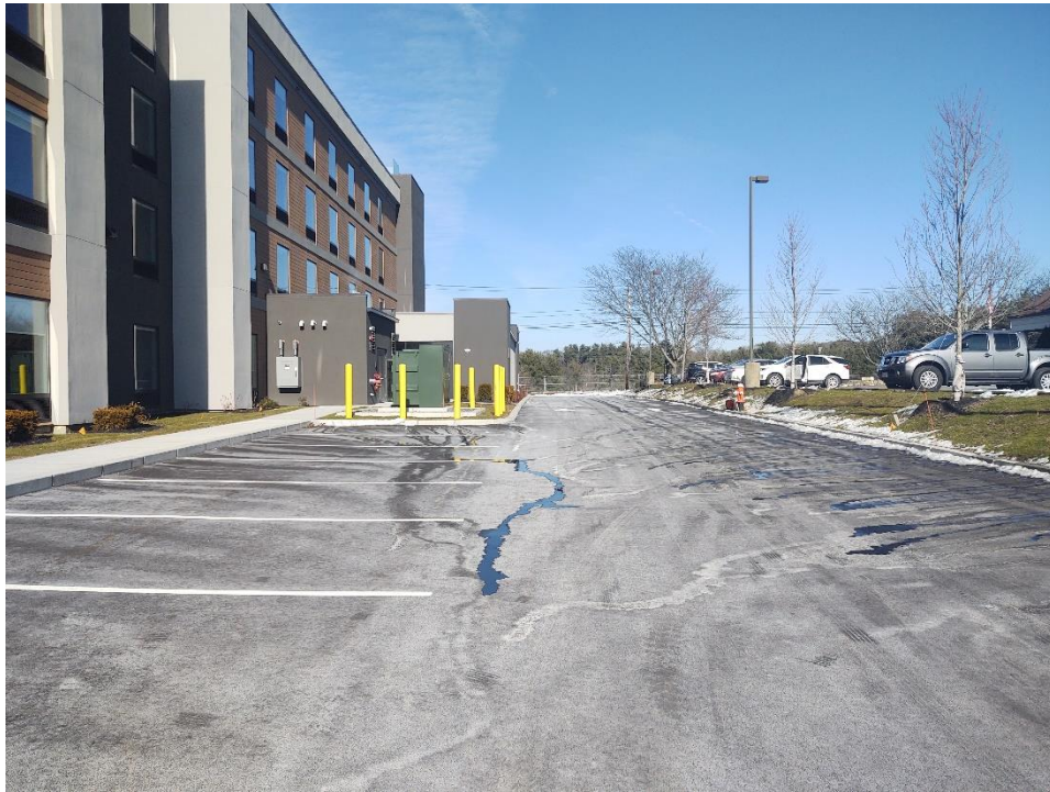
View on east side of building
