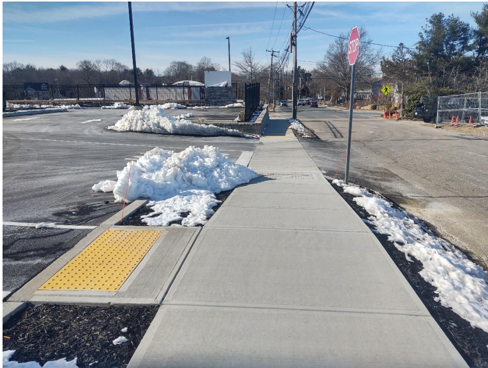
New sidewalk and driveway apron along Union Street
