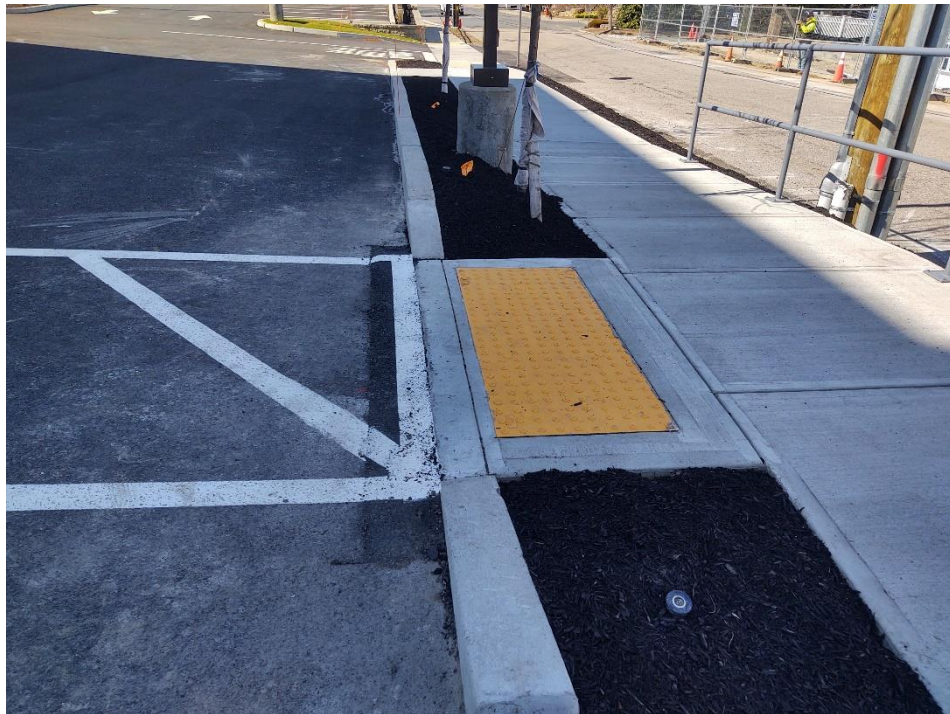
New sidewalk ramp and curb cut
