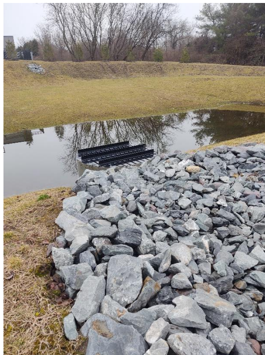
Rip rap reset to proper elevation
