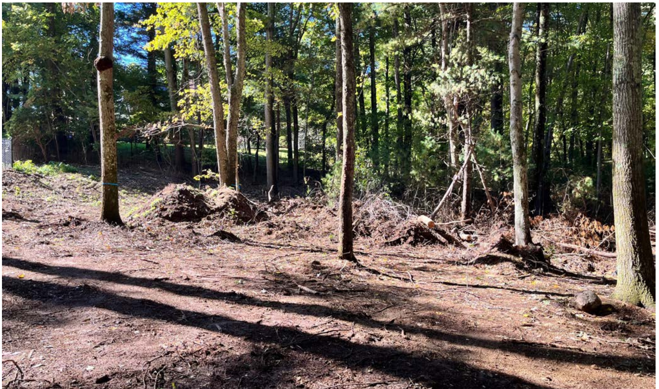
Photo #2: Photo of area of cleared brush with stockpiles.
