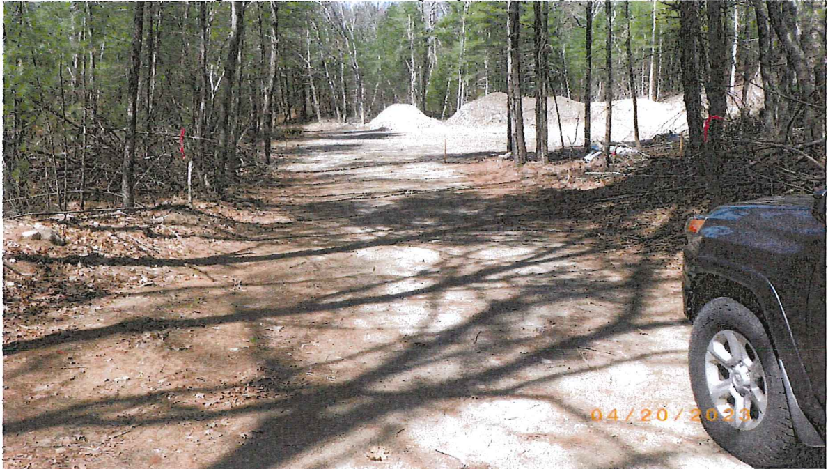
View to site interior along access drive - Pink flags represent "Degraded RFA" Delineation
