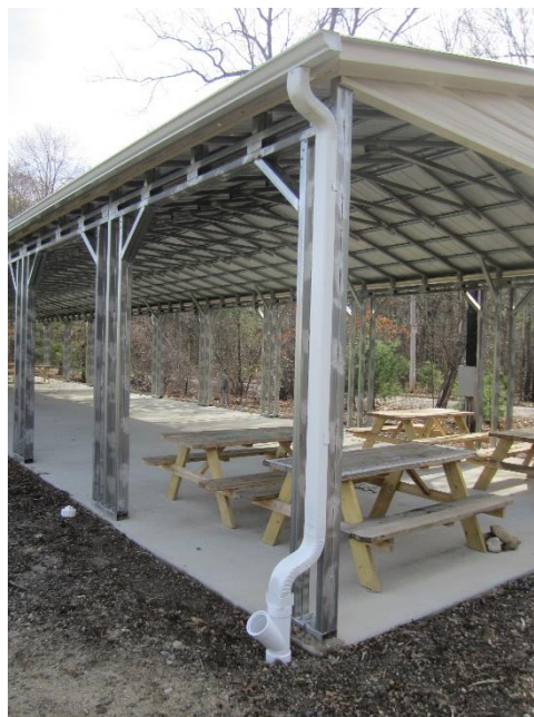
Typical roof leader directed to subsurface infiltration system
