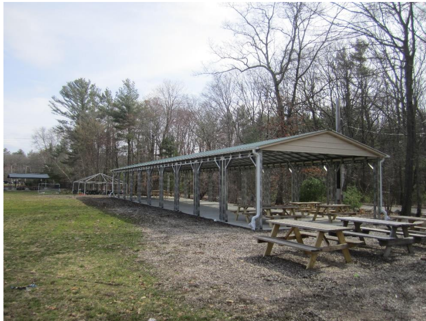
Installed concrete pad with canopy
