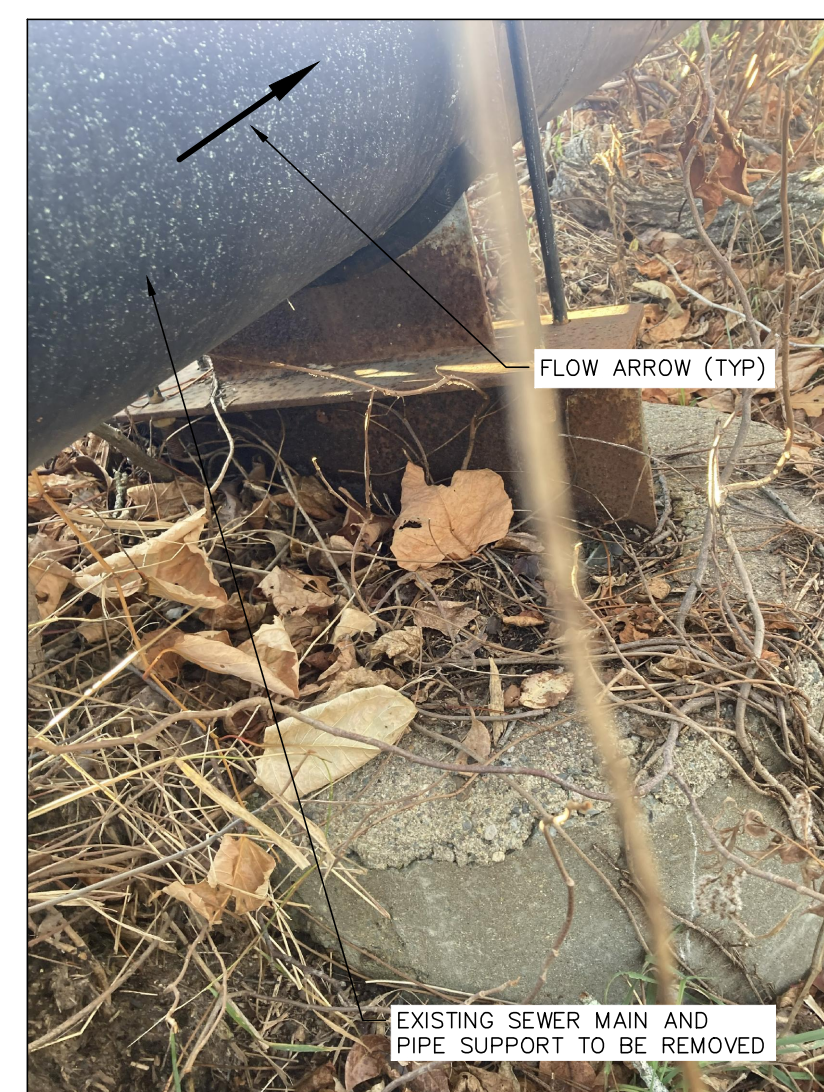
EXISTING SEWER MAIN (APPROX. STA 05+75)
