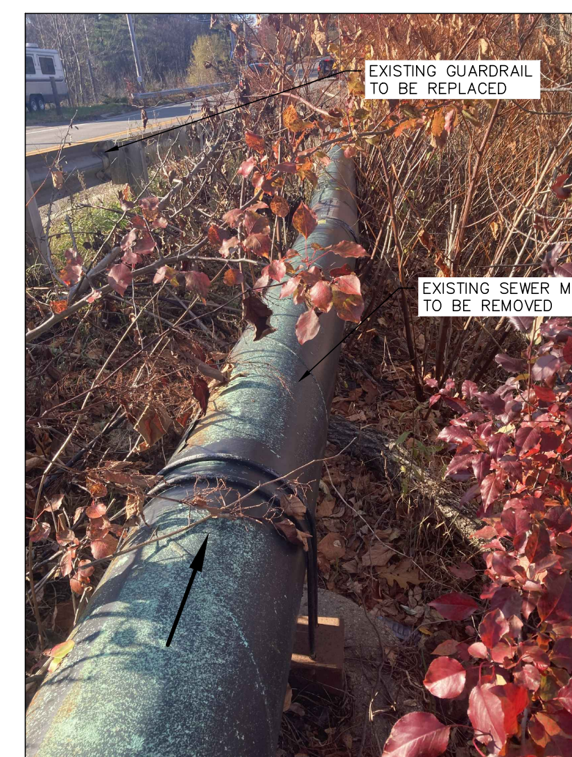
EXISTING SEWER MAIN (APPROX. STA 05+75)
