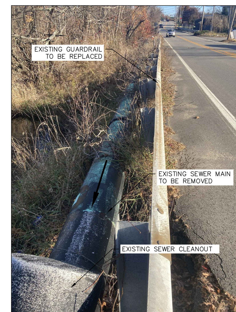
EXISTING SEWER MAIN (APPROX. STA 07+30)
