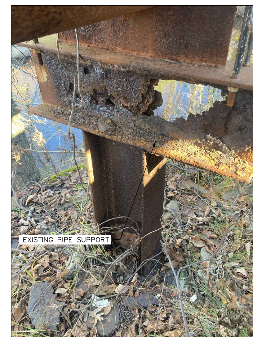
EXISTING SEWER MAIN SUPPORT (APPROX. STA 04+84)
