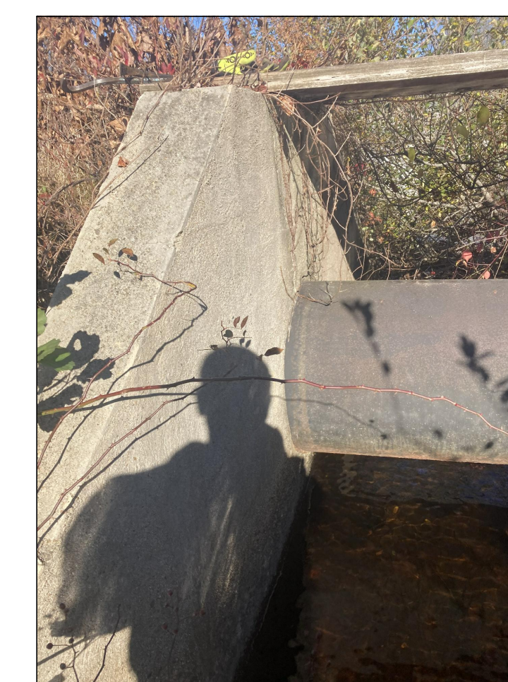
EXISTING EXPOSED PIPE RETAINING WALL TO BE DEMOLISHED
