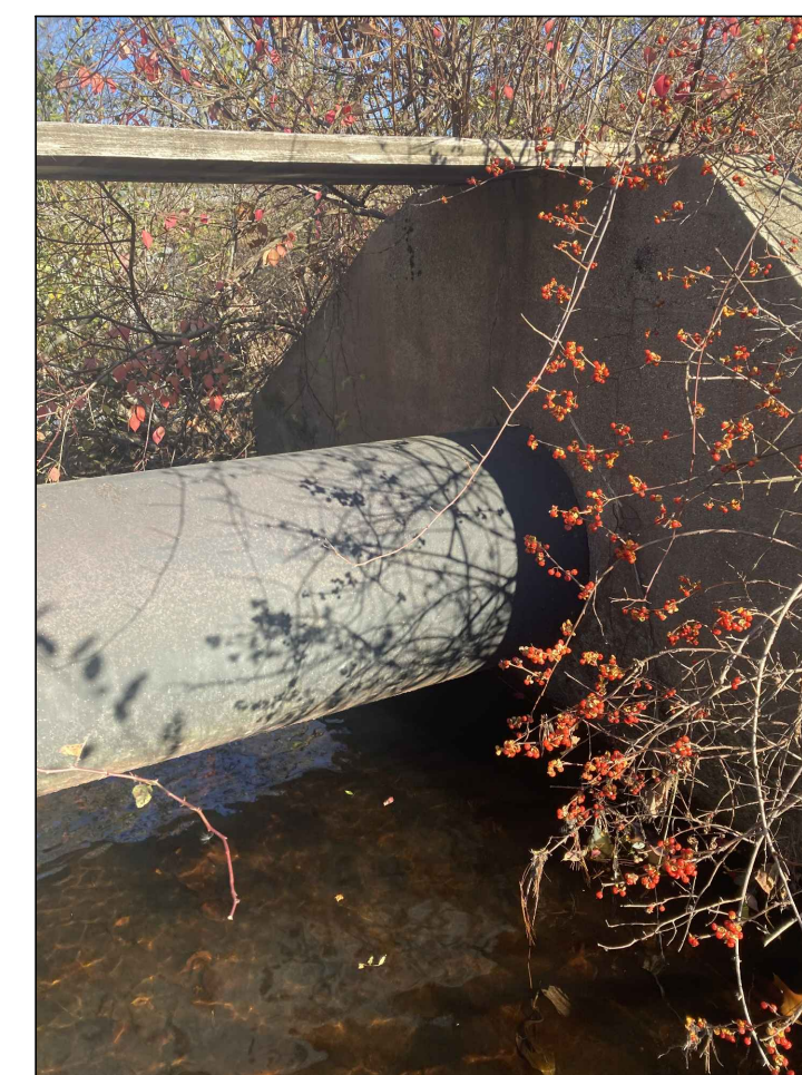
EXISTING EXPOSED PIPE RETAINING WALL TO BE DEMOLISHED
