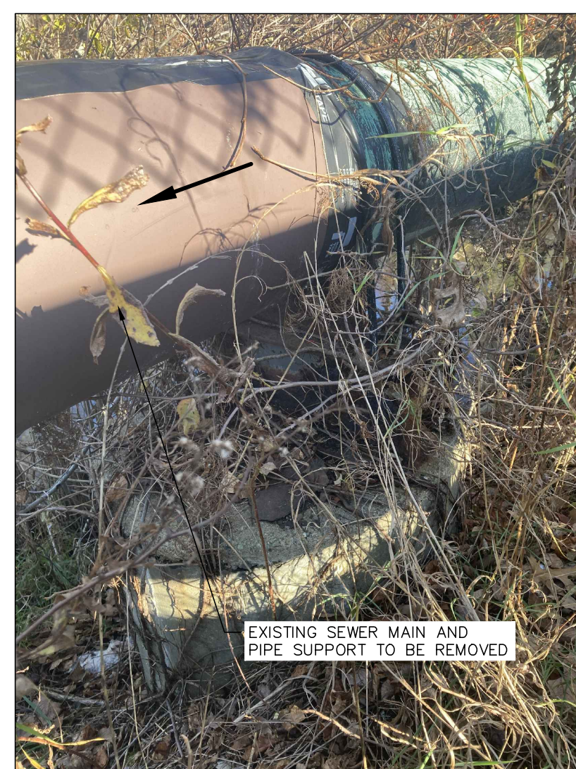
EXISTING SEWER MAIN (APPROX. STA 05+00)
