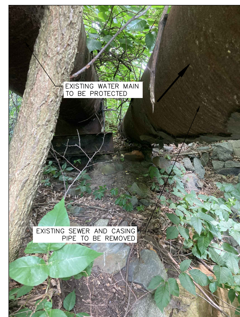
EXISTING WATER AND SEWER MAINS (APPROX. STA 04+35)
