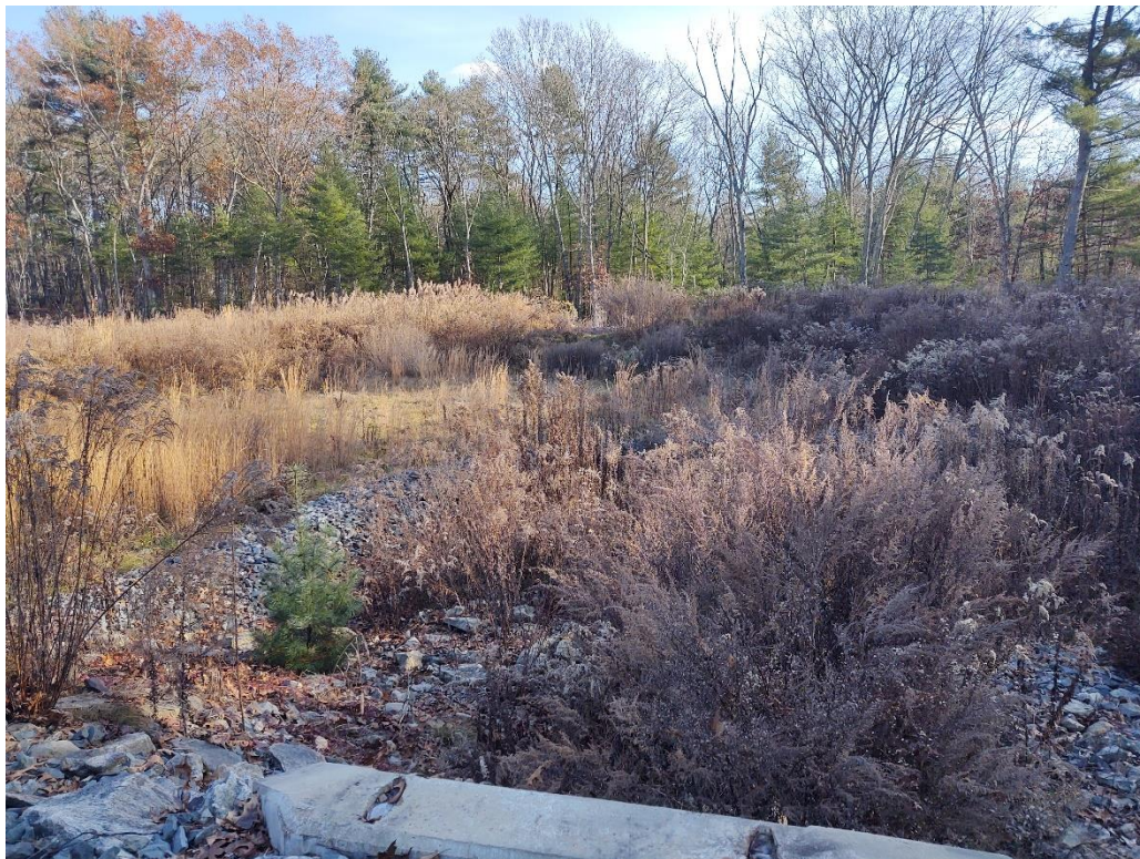
Stormwater basin vegetation
