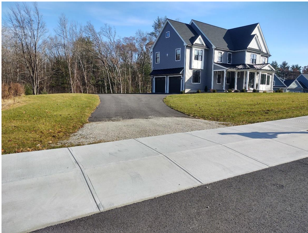
Grading transition at Lot 5-3 driveway
