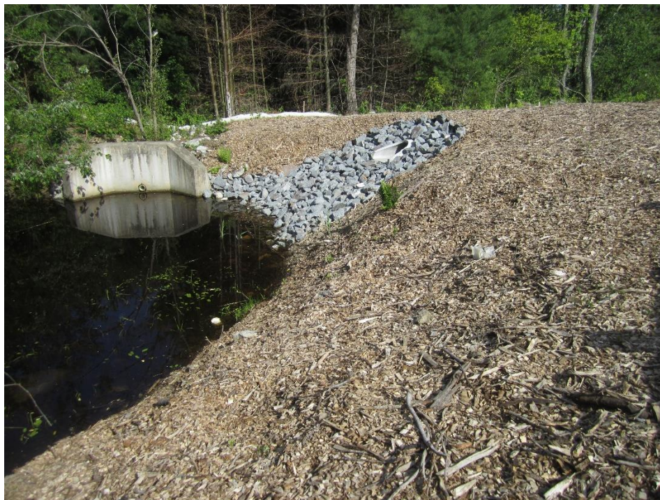
Mulch placement on basin slopes in place of approved "New England Wetmix"
