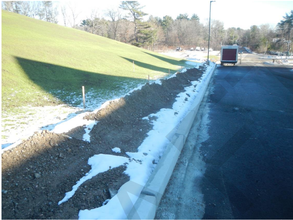
Typical area adjacent to pavement that requires loam and seed installation
