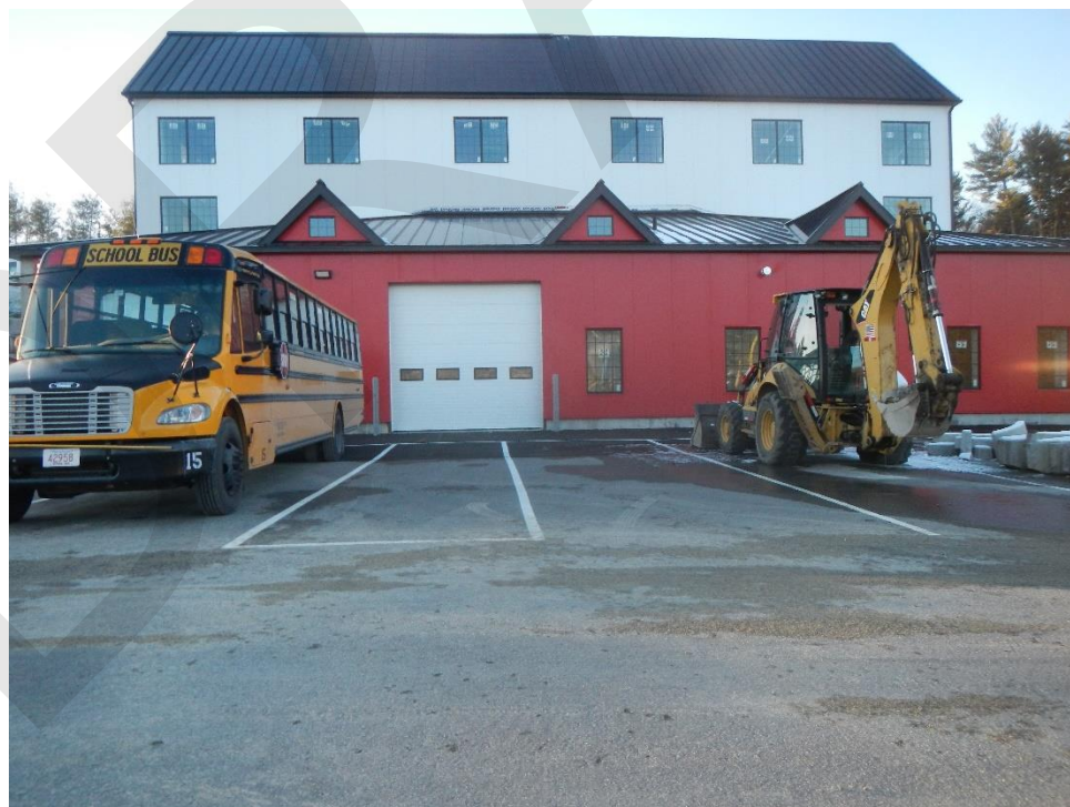
Easterly face of building
