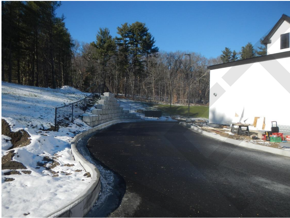
Site driveway near southwest corner of building and retaining wall No. 3
