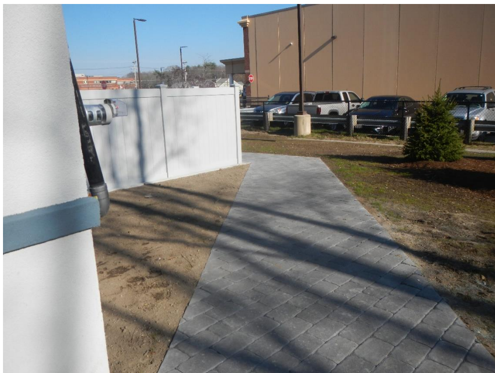
Pervious paver walkway extended from rear of building to dumpster area
