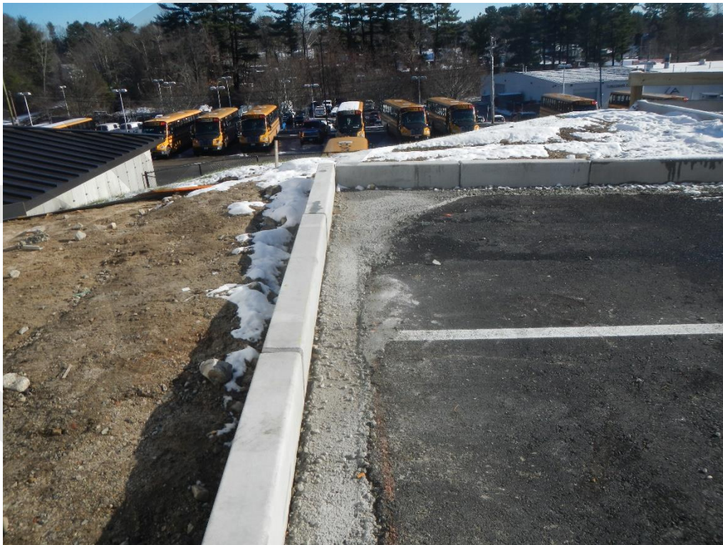
Typical vertical concrete curb installation, locked with concrete
