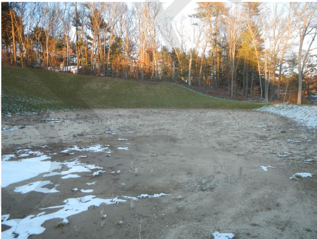
Infiltration basin bottom with no standing water
