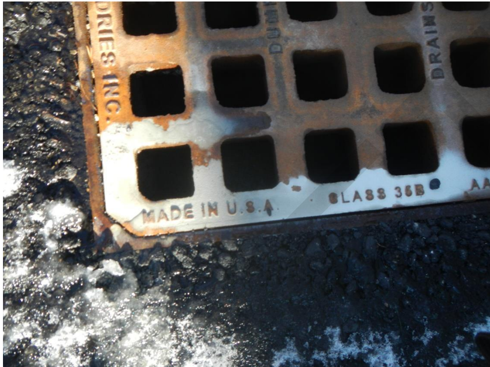
Typical drainage casting meeting Town standards
