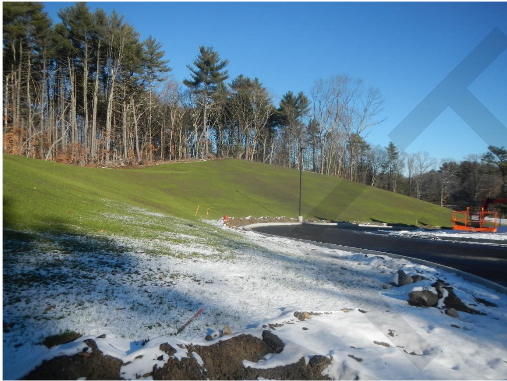
Typical slope stabilized with vegetation
