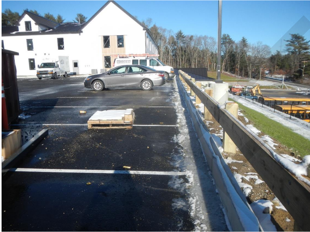
Typical wooden guardrail installation along upper parking area
