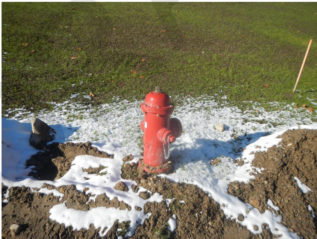
Fire hydrant with orientation towards vegetated slope
