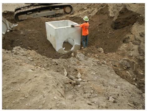
Outlet Control Structure No. 2 with associated outlet pipe, flared end, and splash pad not yet installed
