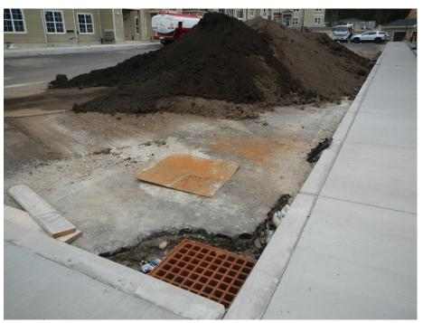
Stockpile areas adjacent to drainage infrastructure without required erosion and sedimentation controls
