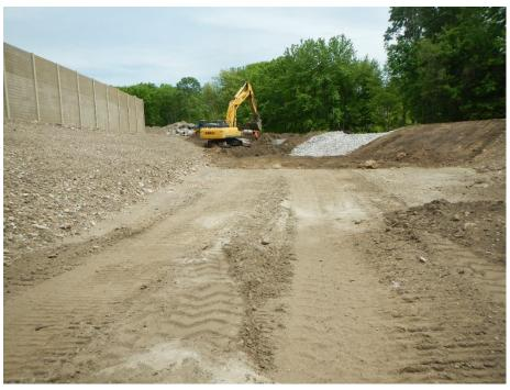
Compacted soils in infiltration basin requiring restoration
