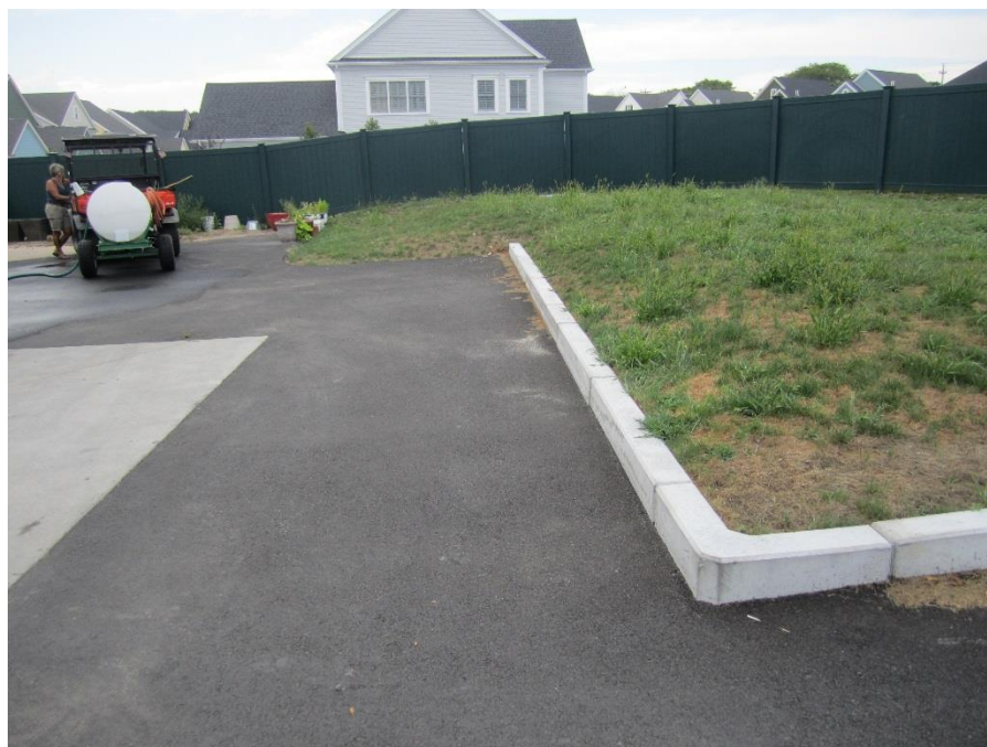
Concrete curb installed in place of concrete apron
