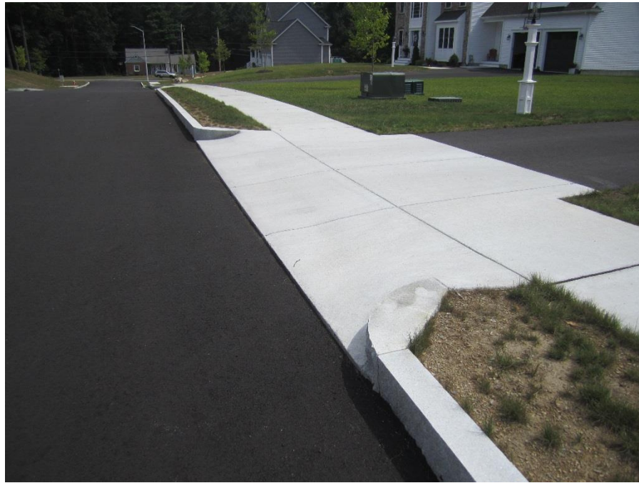
Typical concrete driveway apron
