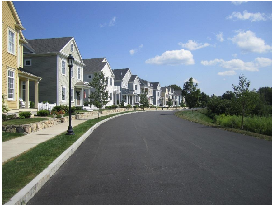
Typical paving (Cooks Farm Road)
