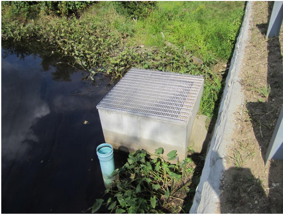
Outlet control structure at Uncas Brook culvert crossing
