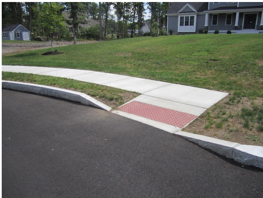
Typical accessible ramp installation
