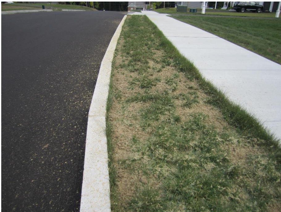
Typical seeding recently done to fill gaps in future Town right-of-way
