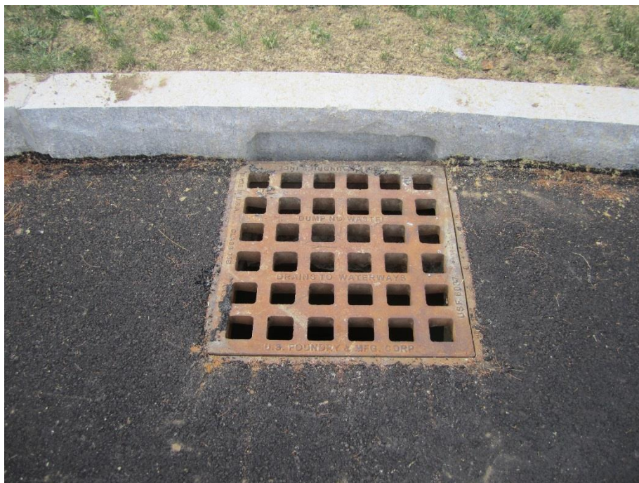
Typical catch basin and curbing
